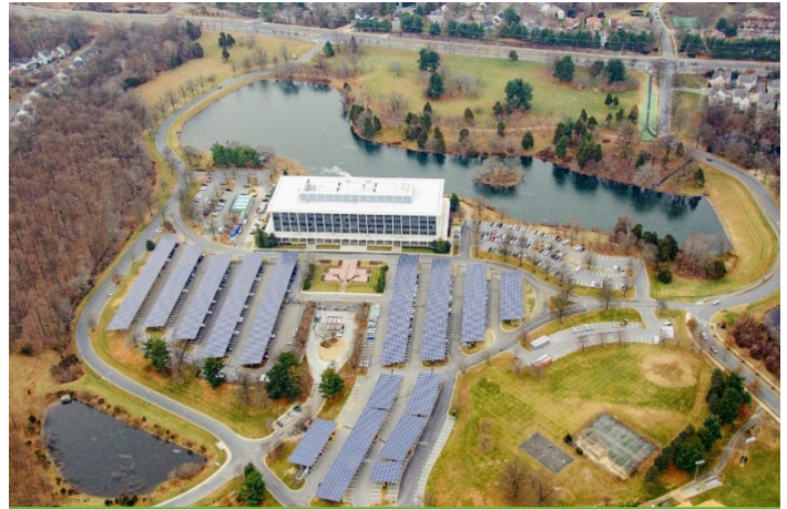
Figure 1. Montgomery County Public Safety Headquarters microgrid. A microgrid serves the Montgomery County Public Safety Headquarters in Maryland with 865 kW CHP, integrated with 2 MW of solar. Find more information at https://chptap.lbl.gov/profile/135/MoCoPublicSafetyHQ-Project_Profile.pdf Photo credit: Montgomery County, Maryland
