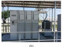
Left: Schematic view of an existing TECO-Westinghouse VersaBridge power converter module system with cabinet that houses the mains controller and three slice cabinets; each cabinet includes three power cubes, an isolation transformer, and slice controllers for the output and active front end controls. Right: A physical installation of a VersaBridge system. Photo credit TECO-Westinghouse Motor Company.
