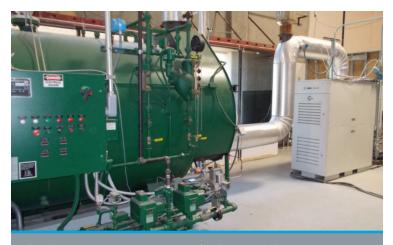
The FlexCHP-65 system consists of Johnston Boiler Company 100-horsepower firetube boiler, GTI-developed supplemental Ultra-Low-NO<sub>x</sub> burner, and Capstone C65 microturbine.
