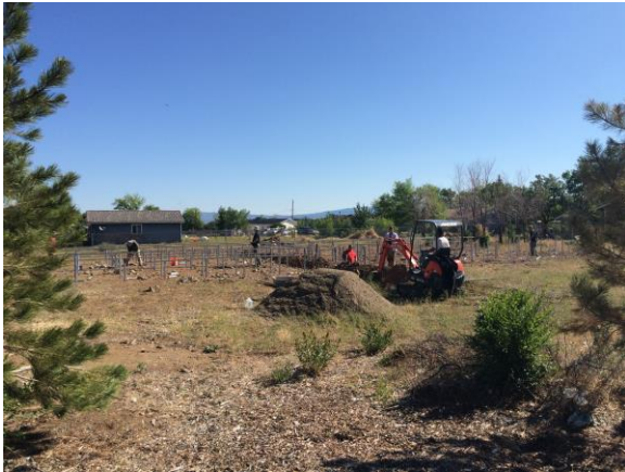
Trench excavation and post installation
