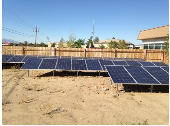
Completed solar array and fencing
