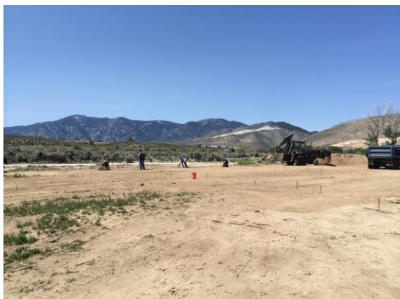
Site grading and staking
