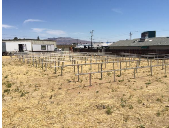
Installation of post and racking system
