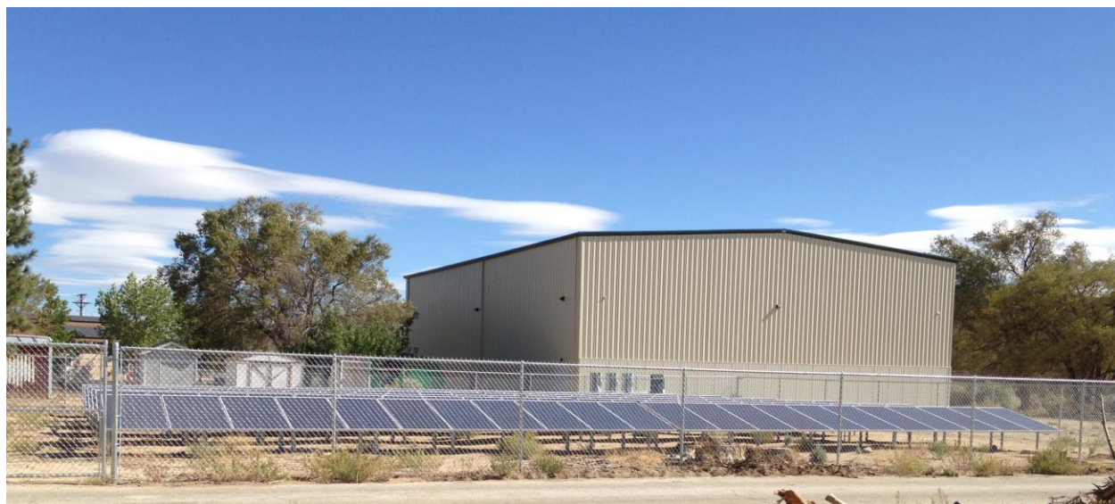
Completed solar array and fencing
