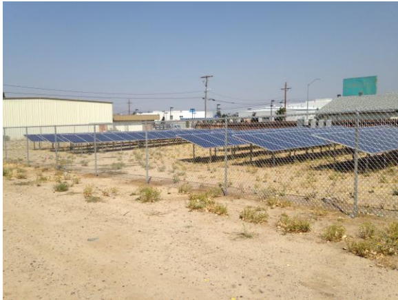
Completed solar array and fencing
