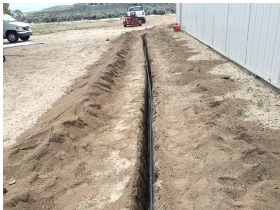
Trenching and laying wire
