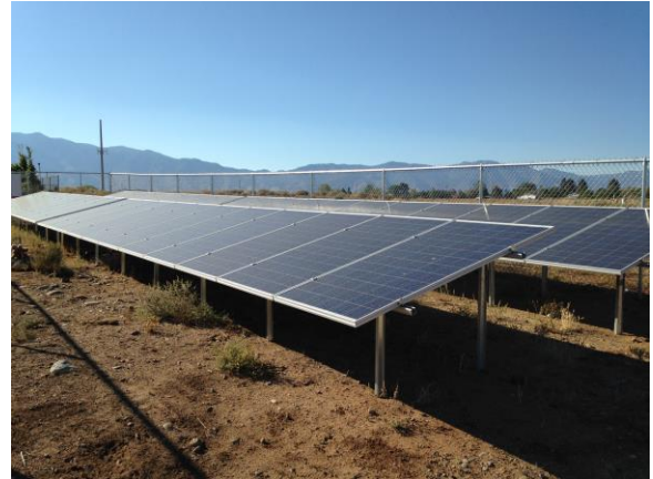
Completed solar array and fencing
