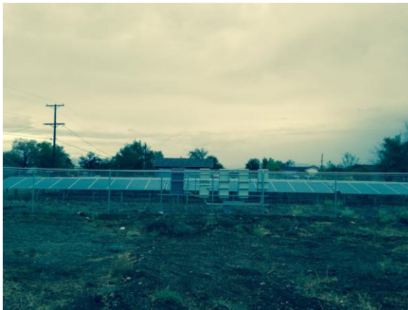
Completed solar array and fencing
