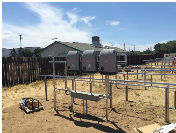
Installation of electrical components box
