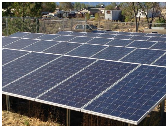
Completed solar array and fencing
