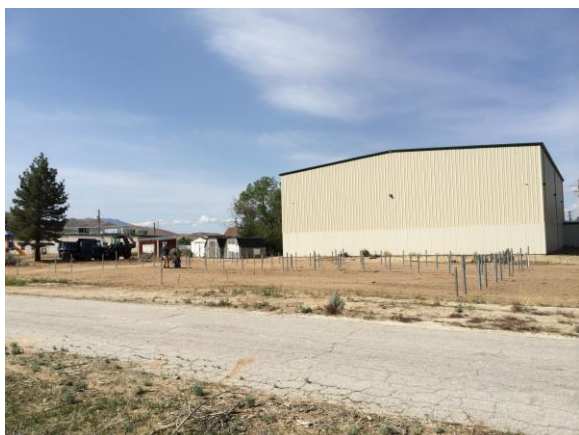
Post and racking installation
