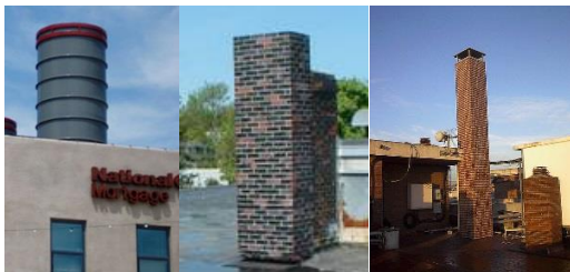
Examples of Roof-Mounted Wireless Communication Facilities (ADD. ORD. 4470 – 3/24/15)
