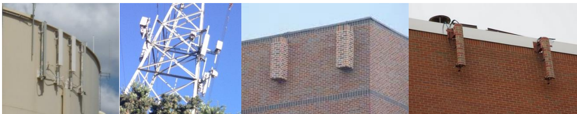
Examples of Flush Mounted Wireless Communication Facilities (ADD. ORD. 4470 – 3/24/15)
