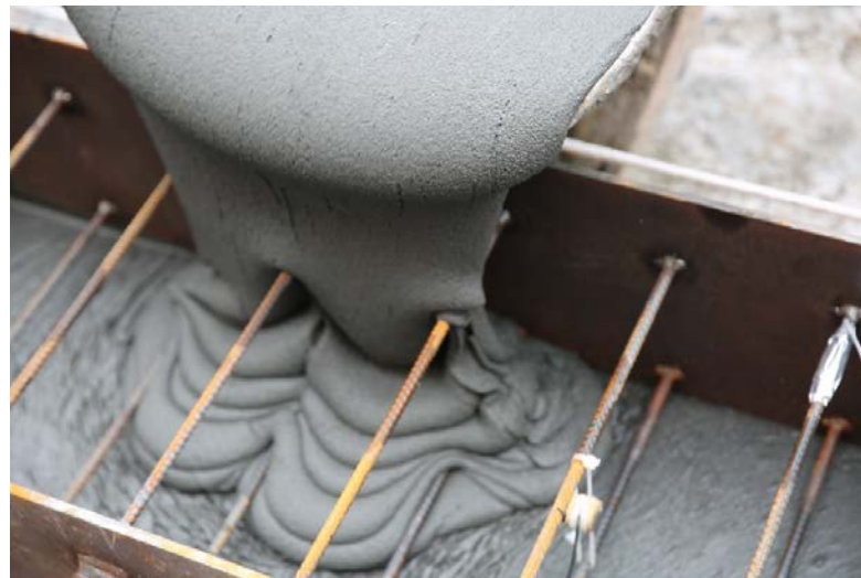
Casting of S-UHPC beam
