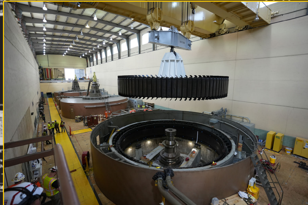
OLD TG, Rotor Removal
