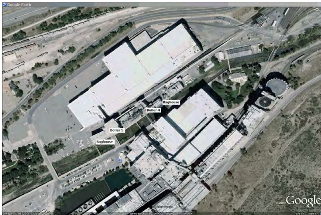
Figure 1: CENC facility Aerial Perspective
