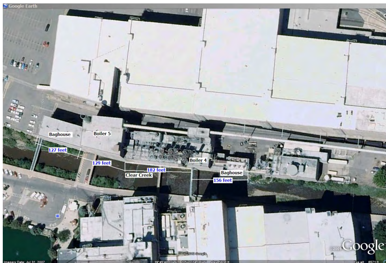
Figure 2: Aerial Zoom of CENC Facility
