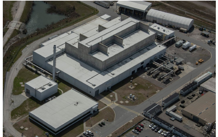
SWPF is processing the majority of the Site's salt solution waste.
