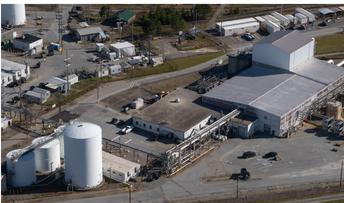
The Effluent Treatment Facility treats low-level radioactive wastewater.
