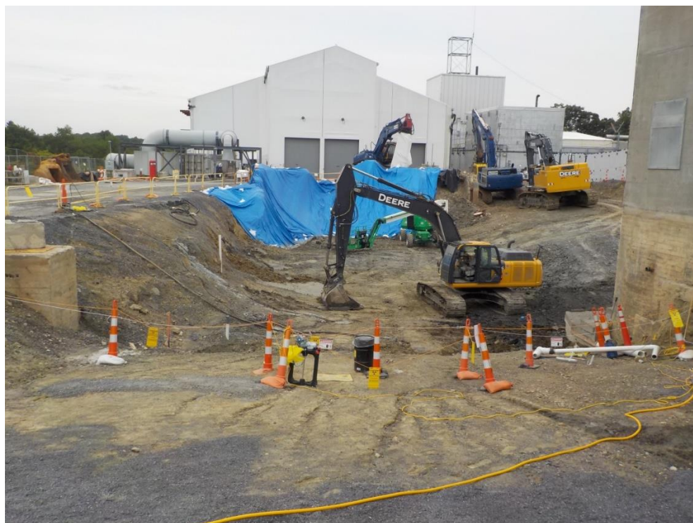
Figure 10. G2 Excavation, Phase 1 (August 29, 2017)
