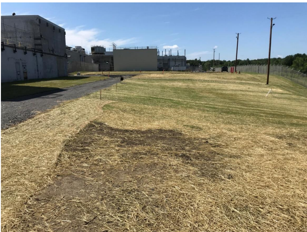
Figure 9. H2 Footprint After Site Restoration (July 26, 2019)
