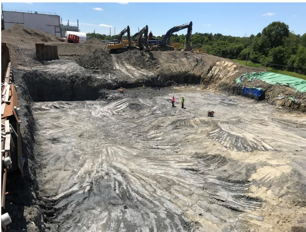
Figure 8. H2 Excavation During Confirmation Sampling (July 21, 2018)
