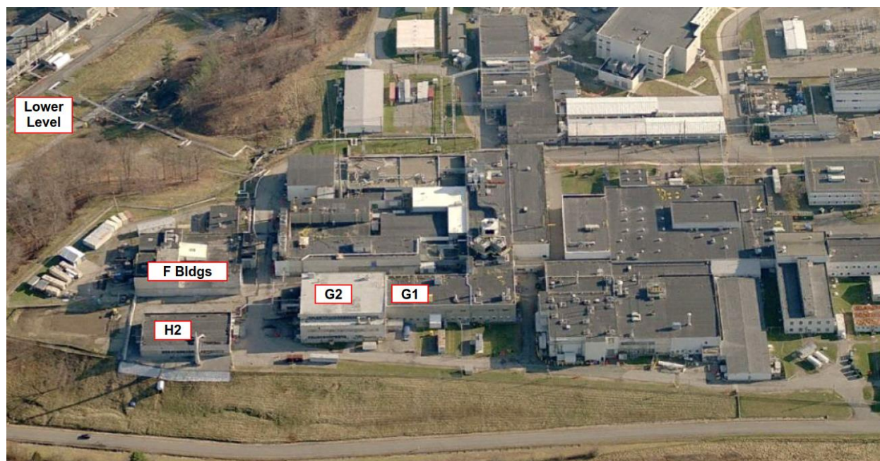
Figure 1. SPRU Site Prior to Decommissioning Project
