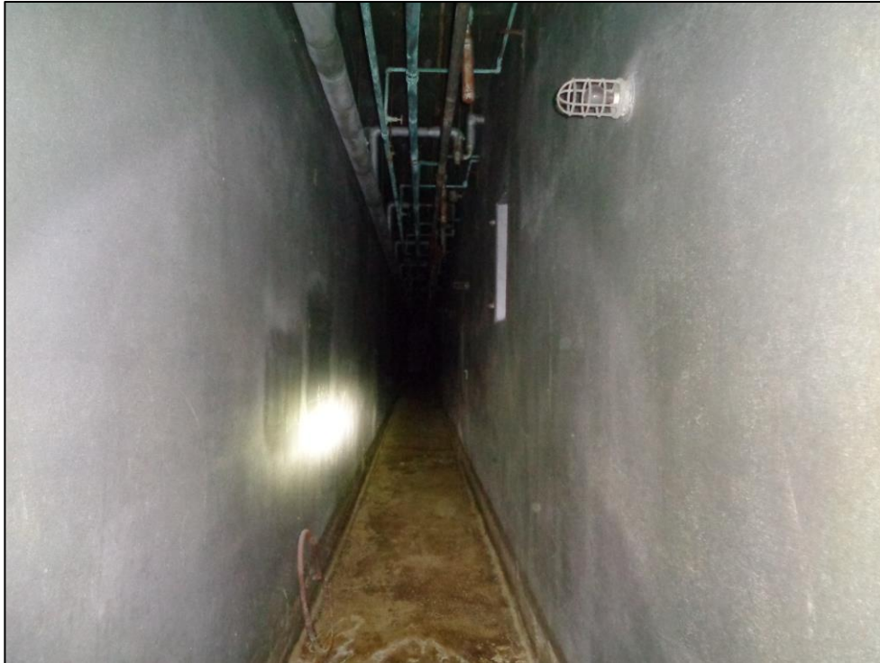
Figure 30. E1 Tunnel prior to decontamination
