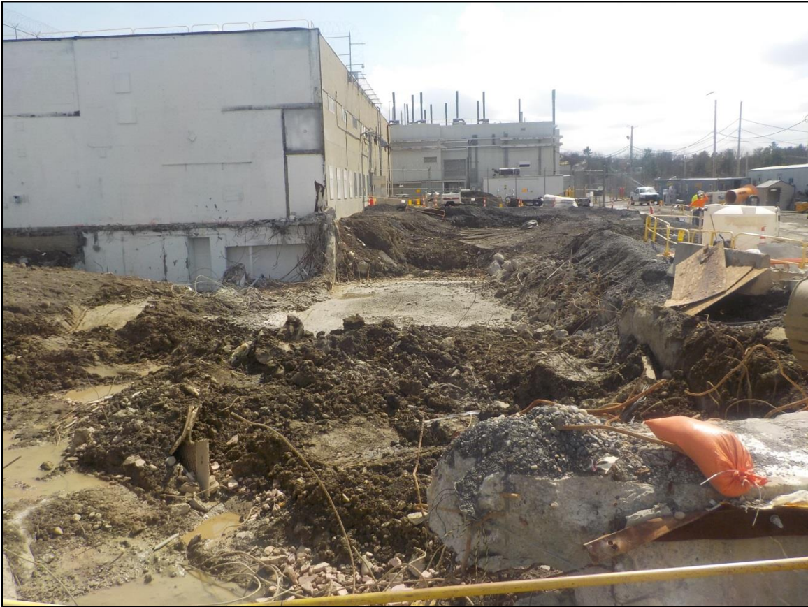
1. G2 area looking south at G1 April 12, 2017
