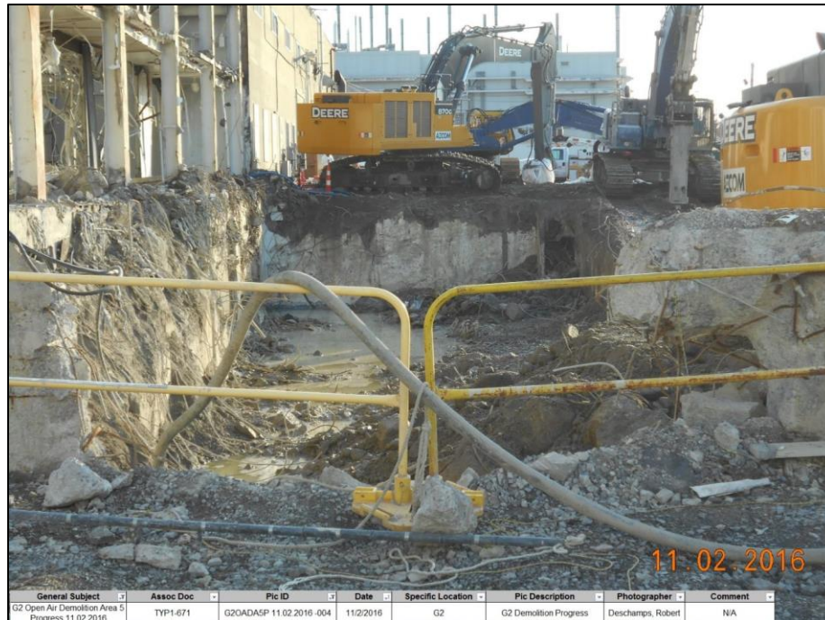
Figure 26. View of the G2 basement after removal of the G2 cells
