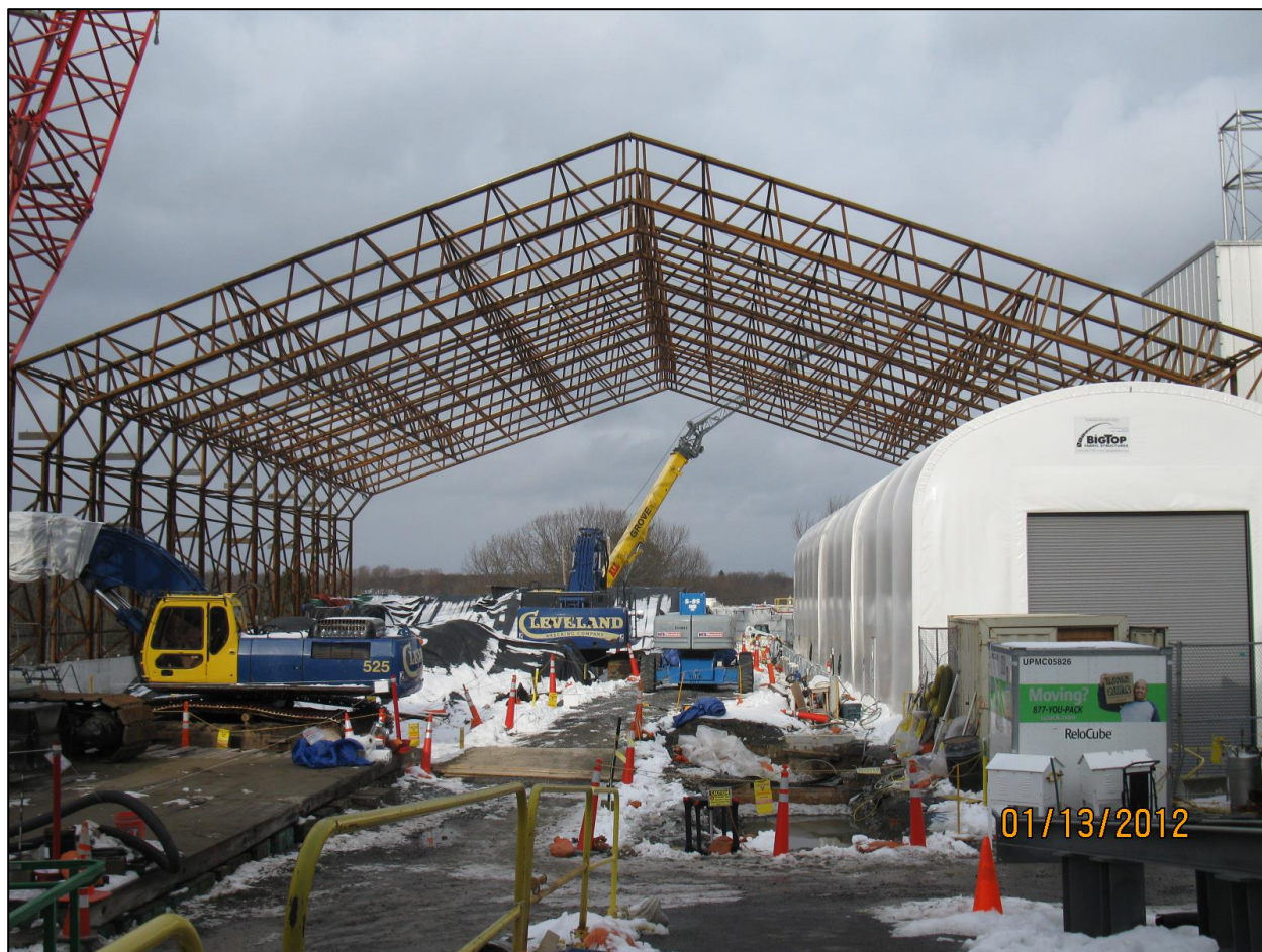
Figure 11. Construction of the steel frame for the H2 enclosure
