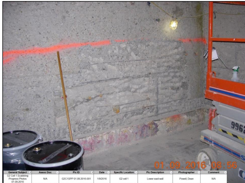
Figure 19. Scabbled walls in empty G2 Cell 1
