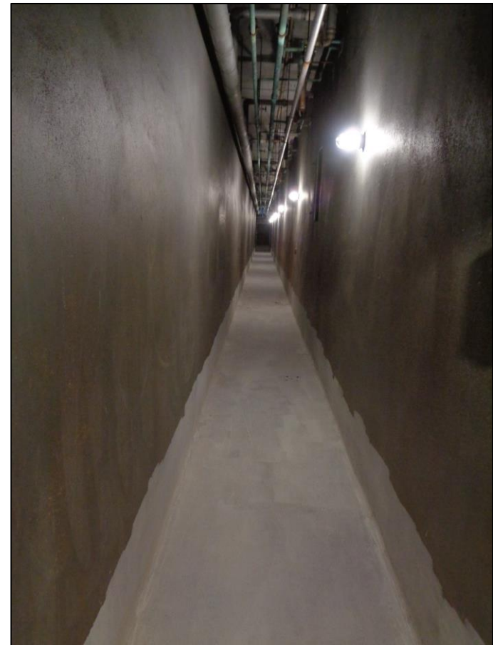
Figure 31. E1 Tunnel post-decontamination
