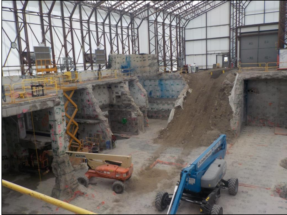
Figure 24. West side of H2 basement after completion of "inside" demolition
