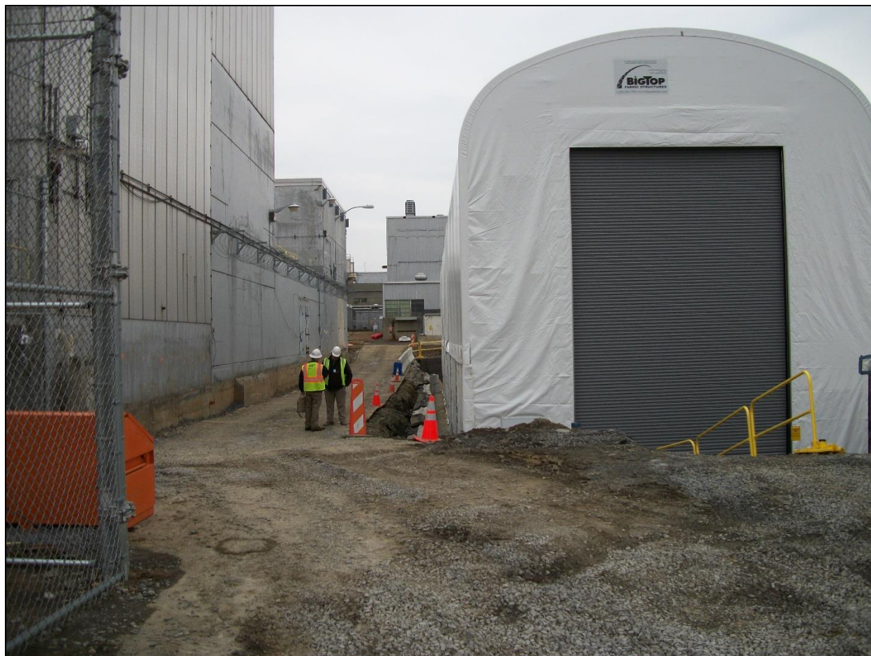
Figure 10 H2 Vault Enclosure (“Big Top”) looking south - March 11, 2010
