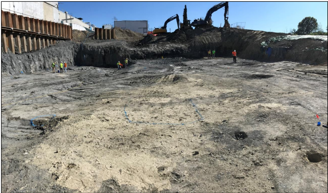
Figure 39. H2 excavation during radiological and chemical verification sampling
