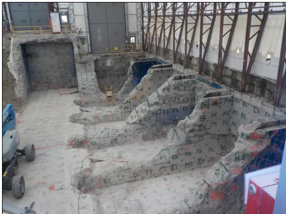
Figure 25. H2 tank vaults ready for open air demolition
