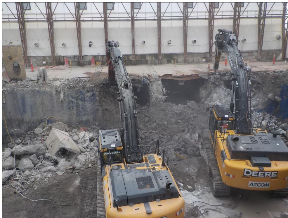
Figure 23. Demolition of H2 tank vaults under enclosure
