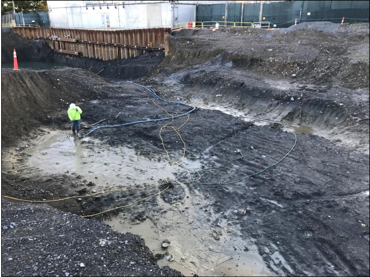
Figure 40. G2 excavation being dewatered prior to backfill
