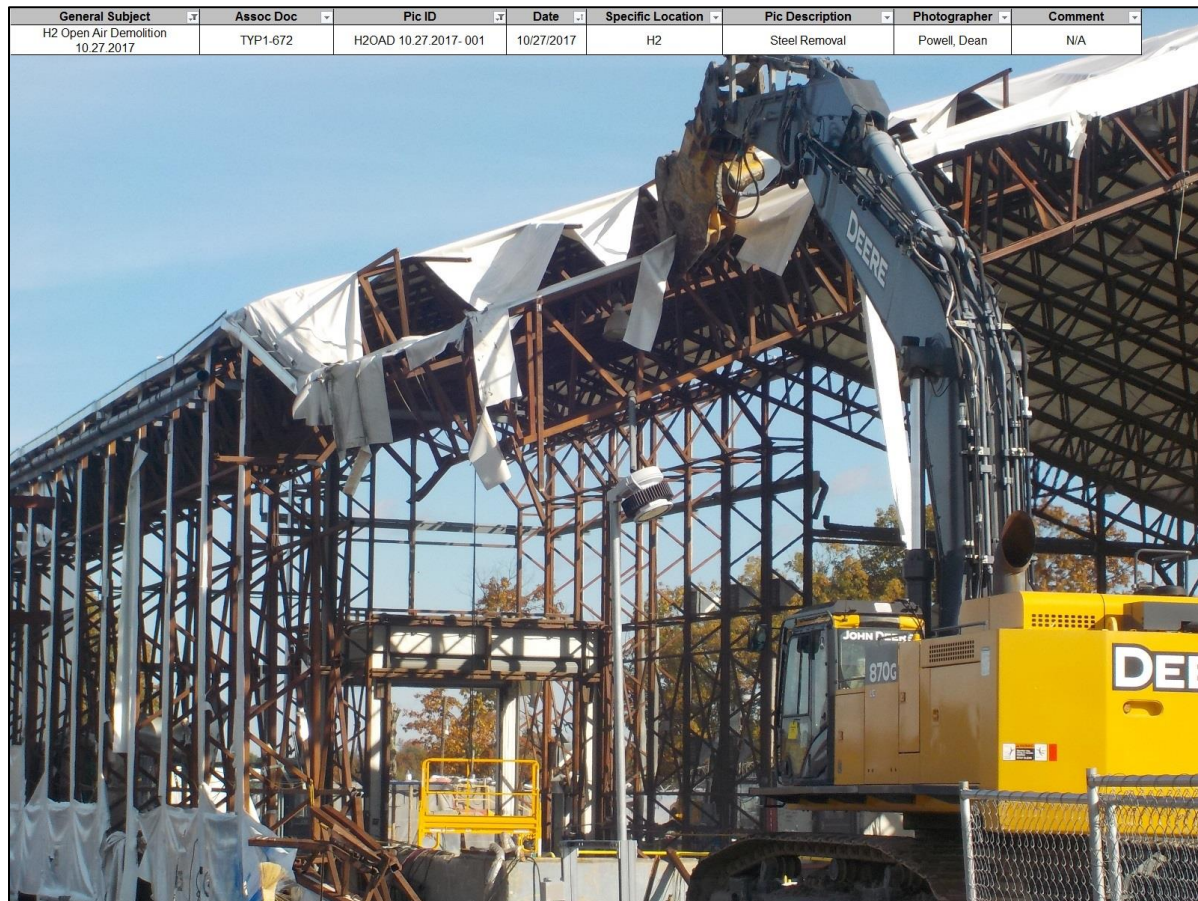
Figure 28. Demolition of H2 enclosure steel frame
