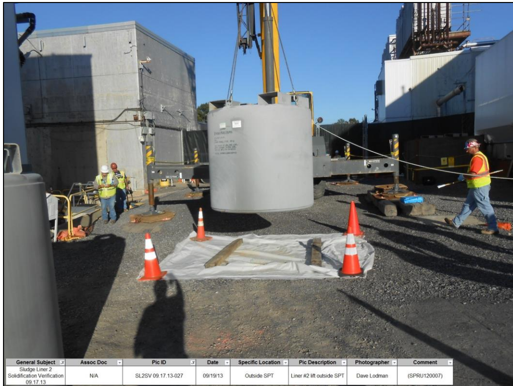
Figure 14. Loaded sludge liner being placed for survey and inspection
