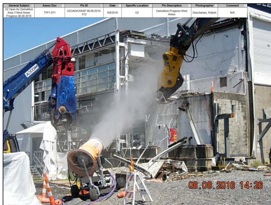
Figure 27. Open air demolition of the west side of G2 using mister for dust suppression
