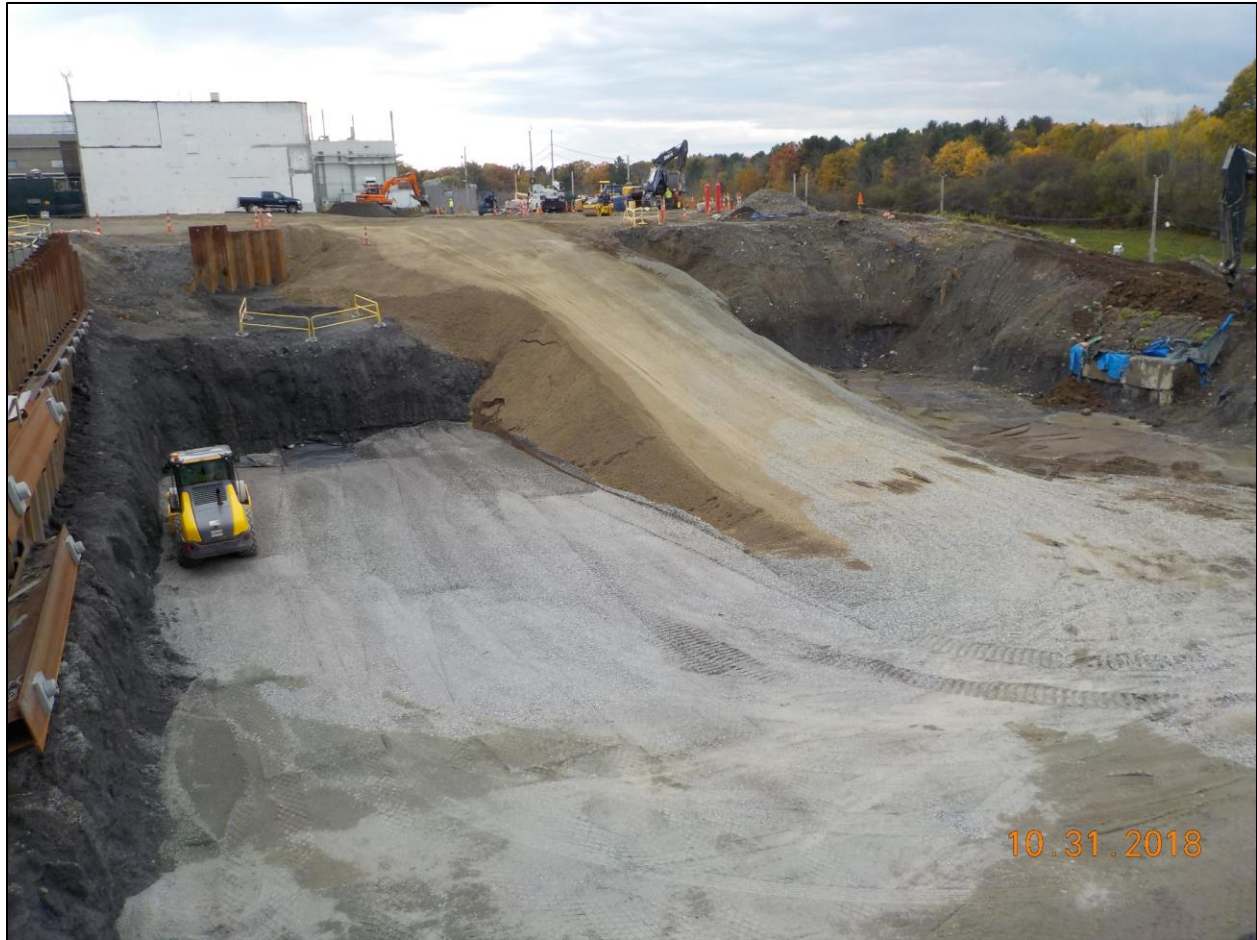
Figure 41. H2 backfill using access ramp from G2 area
