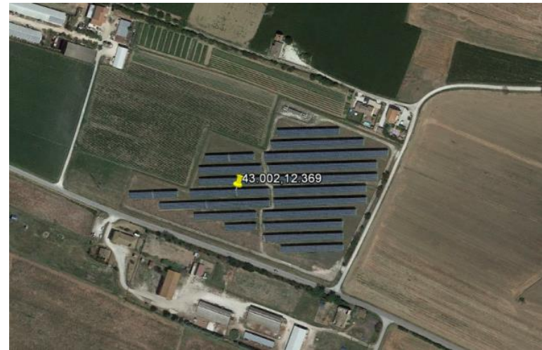
1.935 MW Fixed Array in Italy
