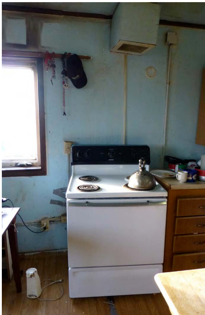
Ventilation fan installed above stove.
