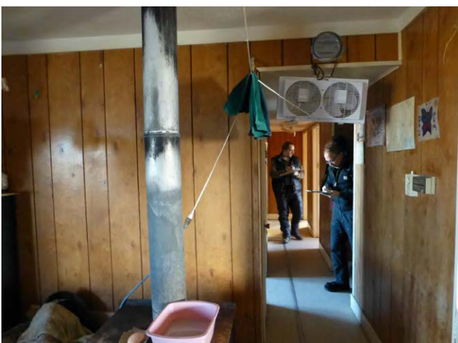
Moses Night House. Occupant has disabled ventilation system but moves warm air through house with fans.
