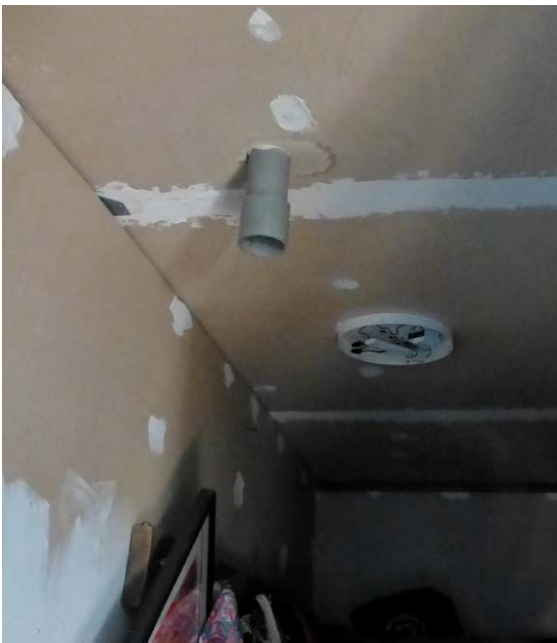
Henrietta Naneng House. A traditional passive vent has been installed in the closet for moist stale air to exit. The building depends on make-up air from the inherent lack of airtightness in the home.
