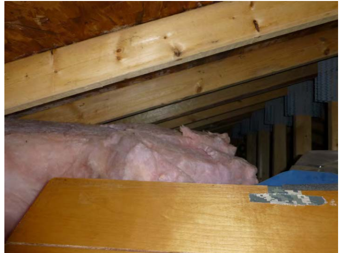
The cold roof with 8" of bat insulation and hatch into main living area
