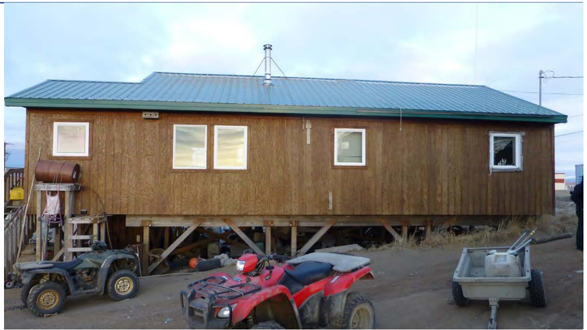
The house has experienced some settlement, but the foundation is not adjustable by occupant.
