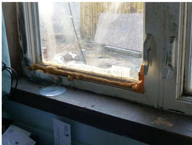
The windows are poorly caulked and drafty. The occupant covers them with plastic in the winters.
