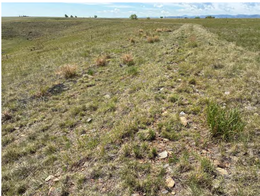
Figure 4. Looking South-Southeast at a Diversion Berm that Runs Along the Eastern Pediment, Which Was in Good Condition
