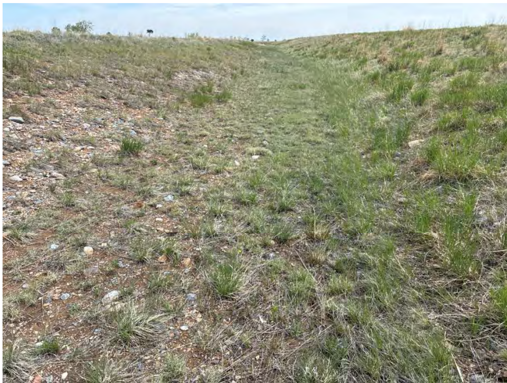
Figure 5. Looking Northeast at the Northern Vegetation-lined Perimeter Channel, Which Was in Good Condition
