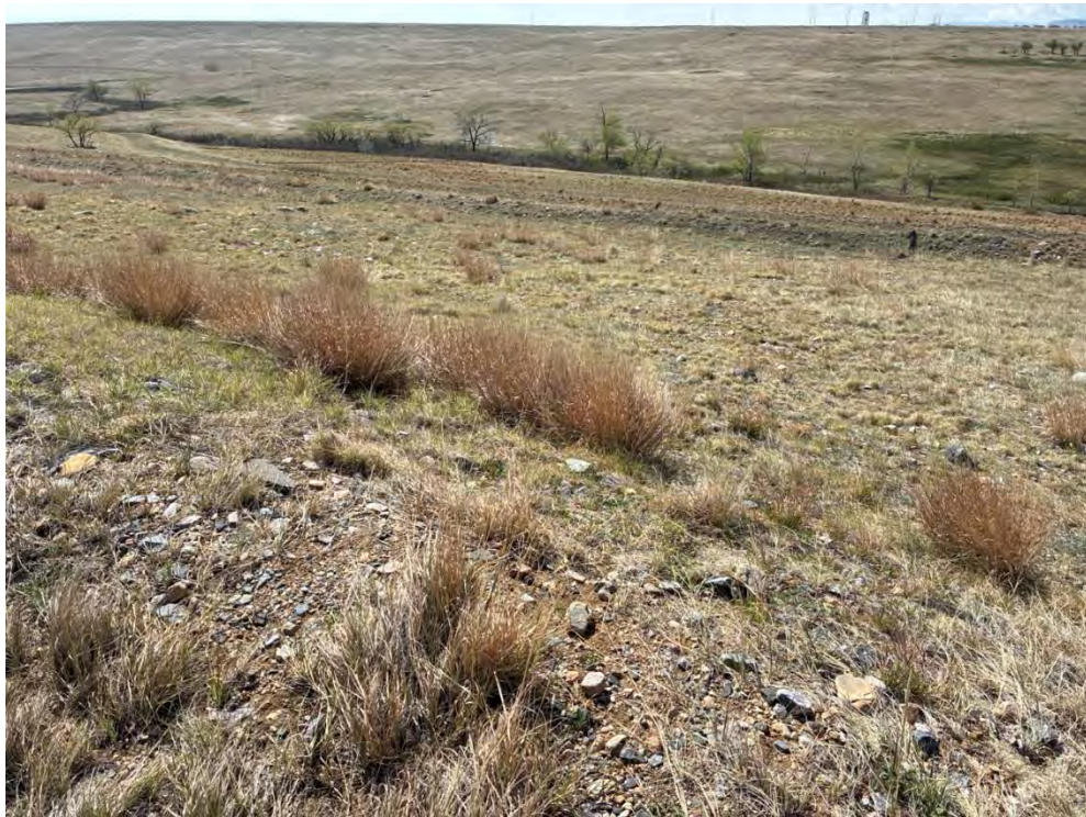
Figure 5. View Looking Southeast at Berms 4–7, Which Were in Good Condition
