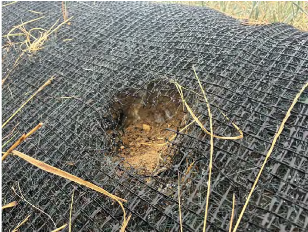
Figure 4. View Looking East at Berm 3, Where a Small Mammal Hole Was Noted
