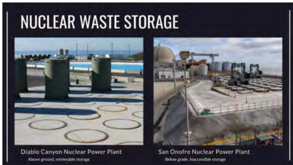
This image demonstrates the difference between the above ground storage system and the partially below grade system.
