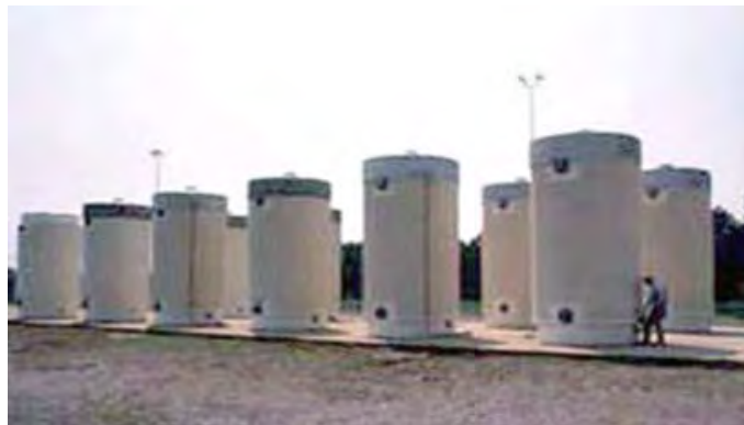
Fig. 4. View of large vertical DSCs containing HLW.
