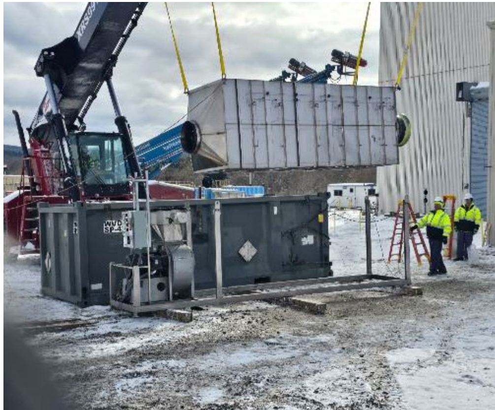
Loading the first RVU into a waste container
