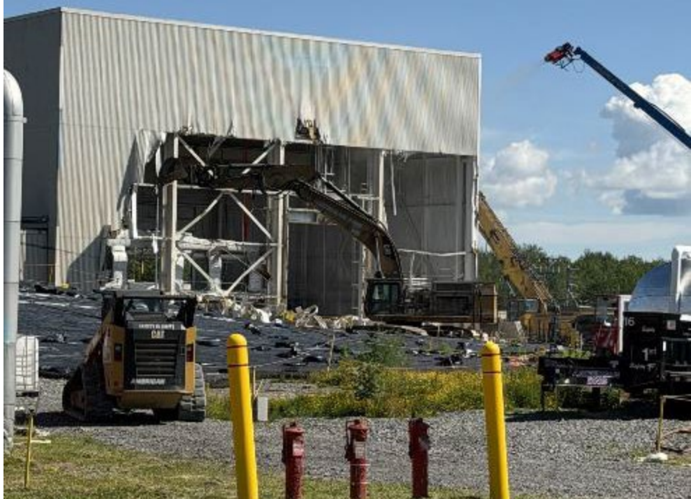
The start of deconstructing the FRS
