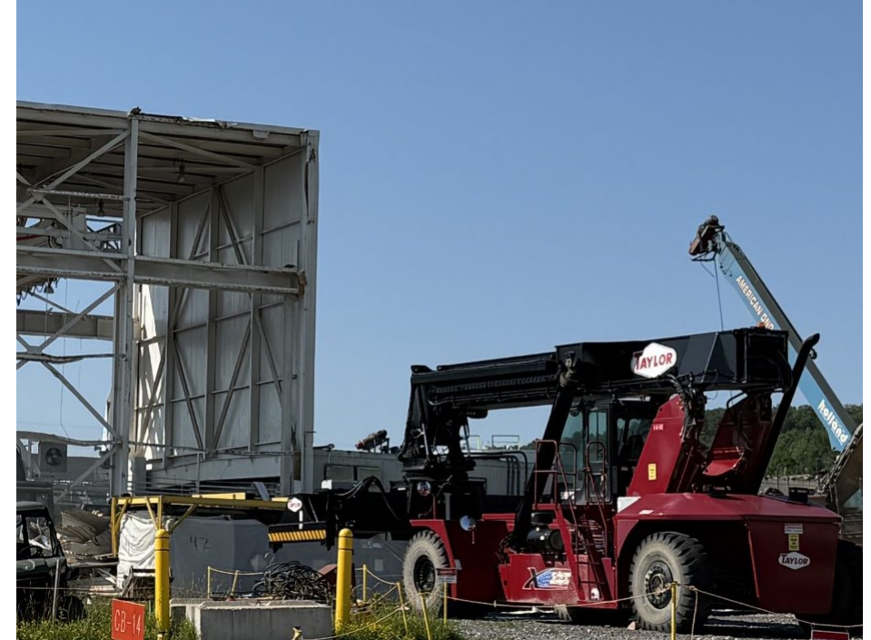
A reach-stacker places an empty waste container inside the FRS work area
