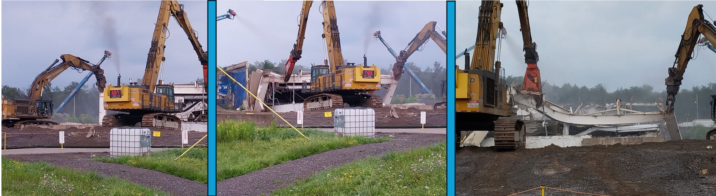
Taking down the FRS lower bay structure
