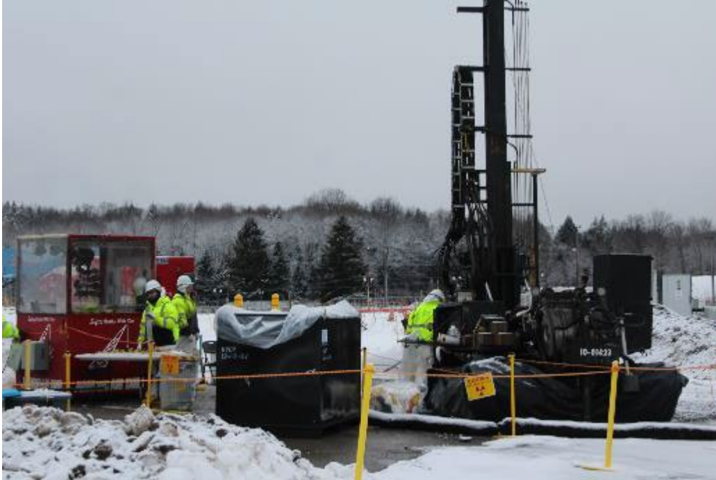
Retrieving samples to characterize the soil for constructing a retention wall (needed for excavation)
