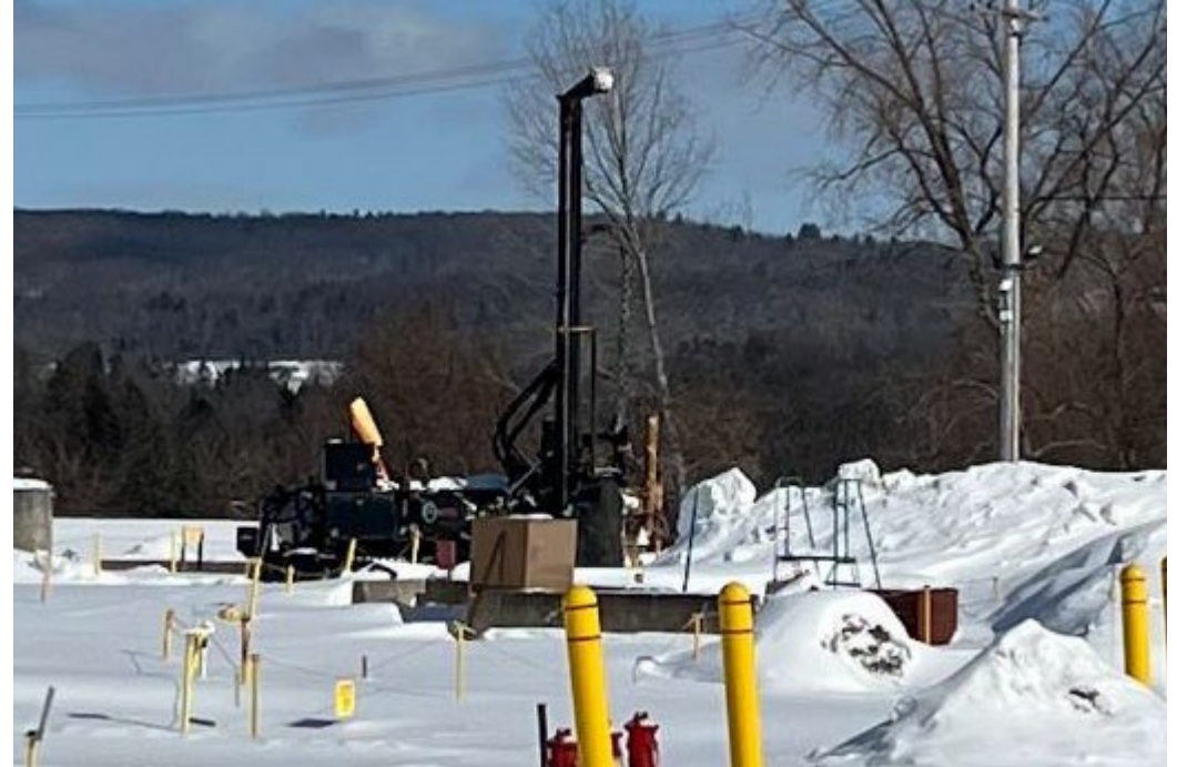
Workers completed 19 of 20 geotechnical borings and 4 of 5 piezometer installations, equipment being demobilized
