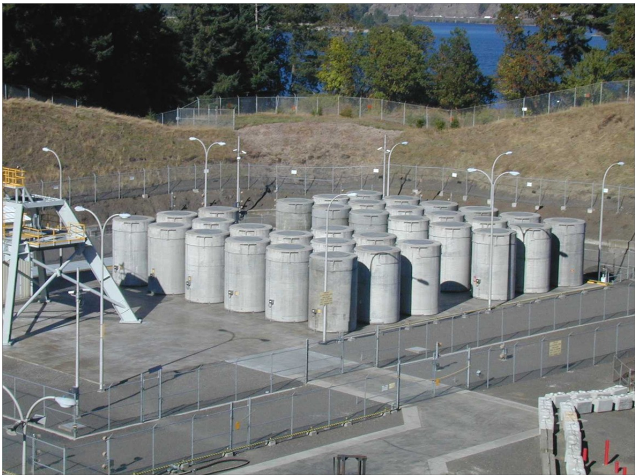
Figure 2-22. Trojan Independent Spent Fuel Storage Installation
