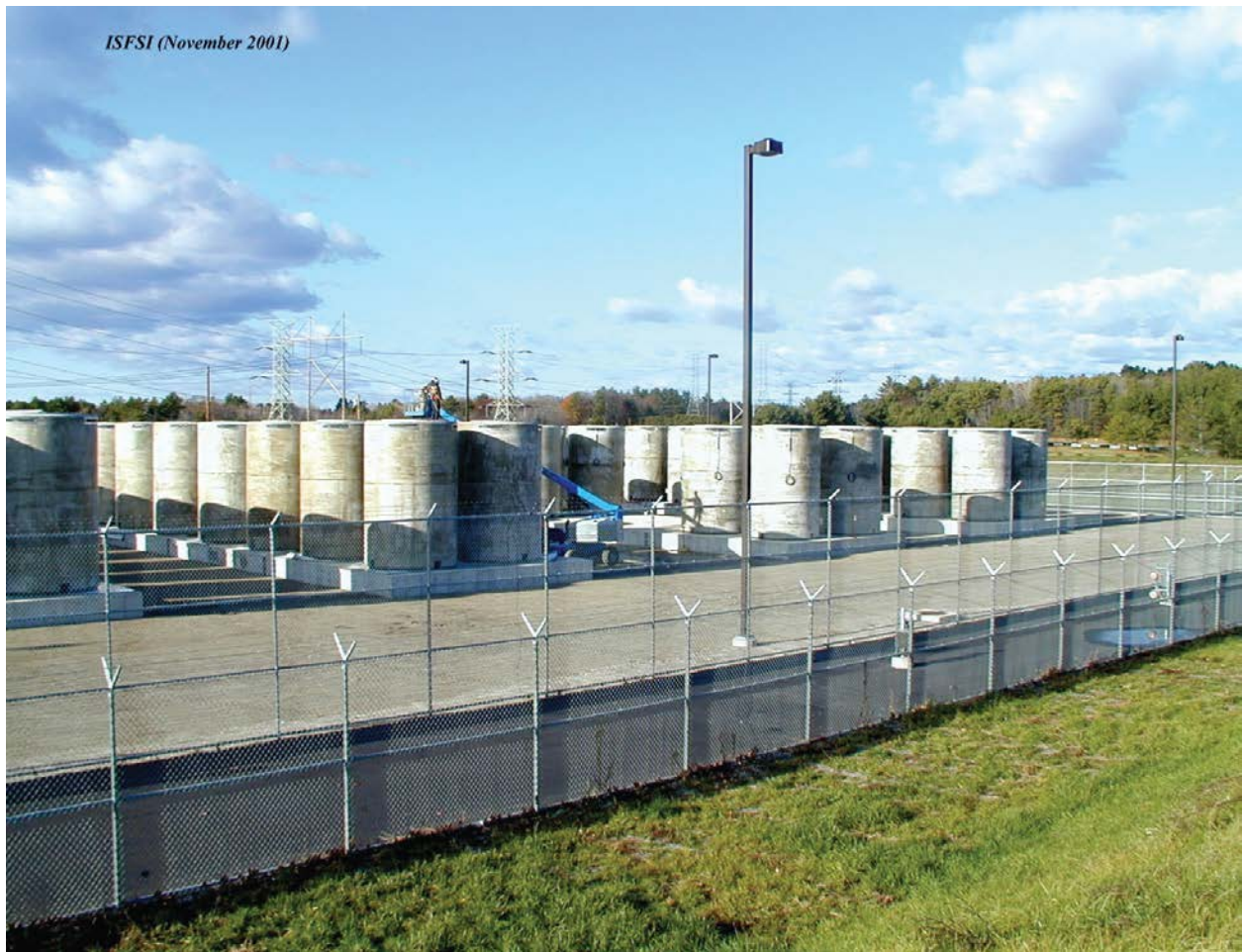
Figure 2-4. Maine Yankee Independent Spent Fuel Storage Installation
