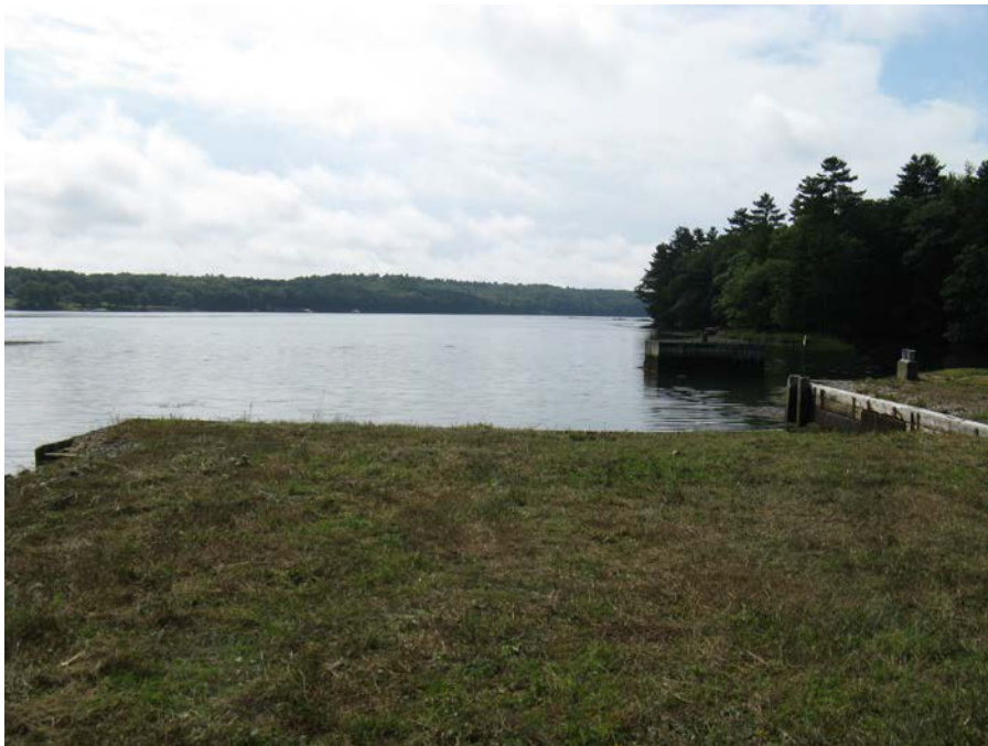
Figure 3-4. Barge Dock at the Maine Yankee Site
