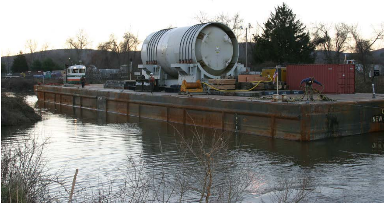
Figure 2-38. Connecticut Yankee Reactor Pressure Vessel Being Transported on Barge
