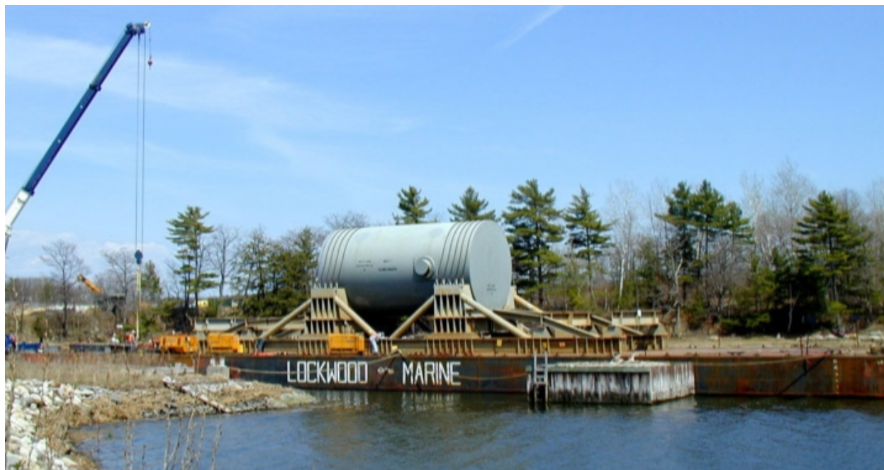
Figure 2-15. Maine Yankee Reactor Pressure Vessel Being Loaded onto Barge
