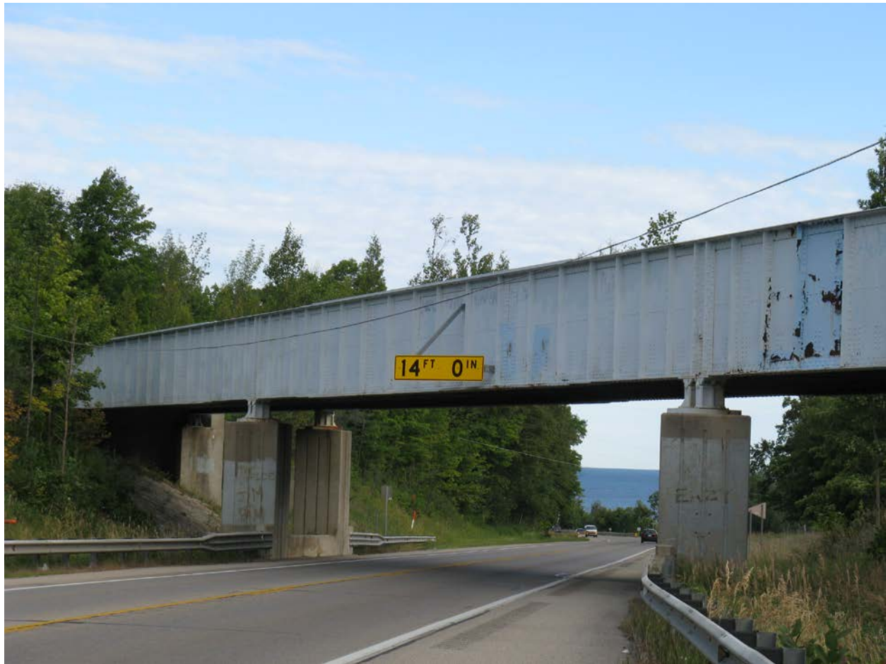
Figure 2-67. Low Overhead Clearance Abandoned Railroad Bridge
