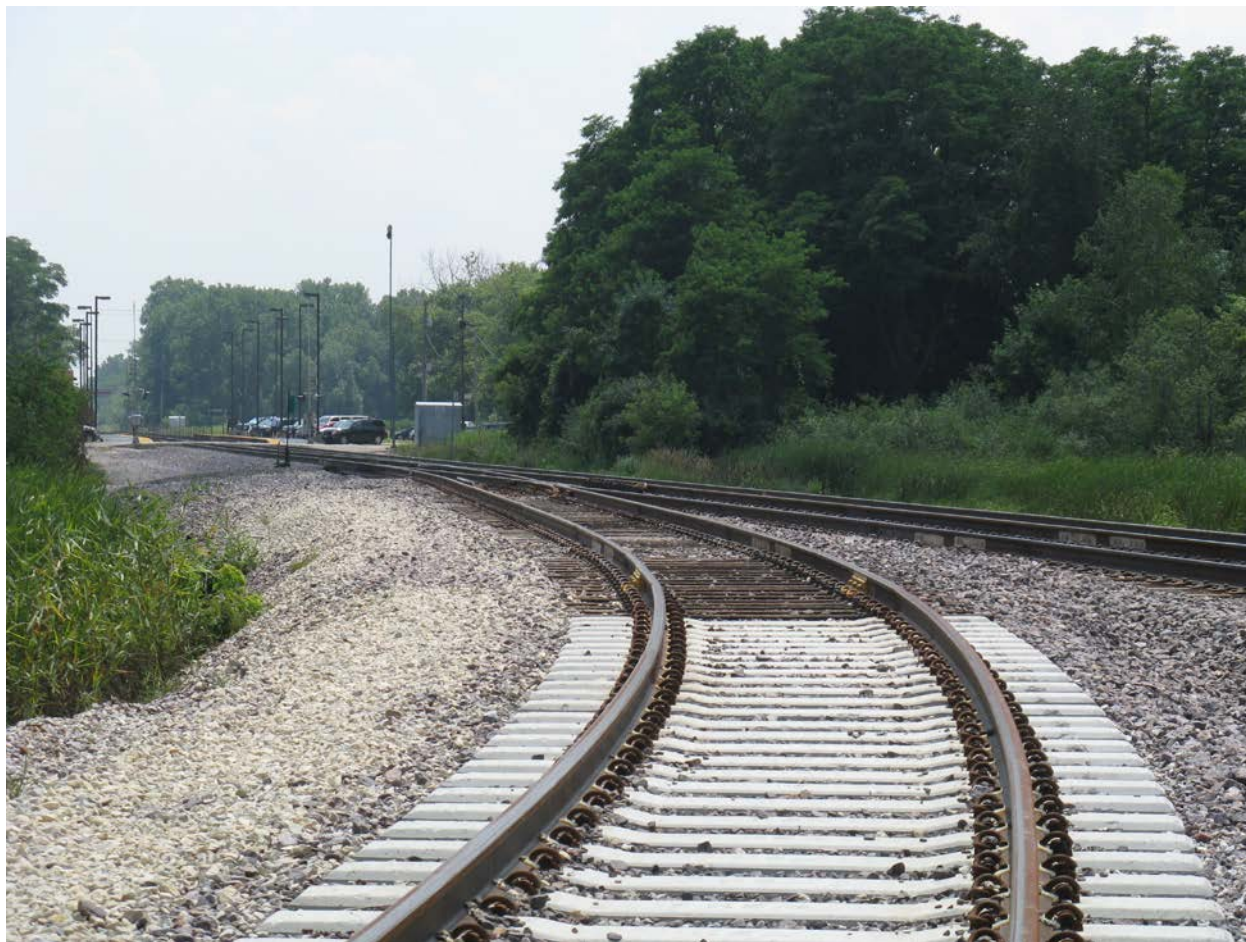
Figure 2-124. Junction of Zion On-site Rail Spur with Union Pacific Railroad Showing Concrete Rail Ties
