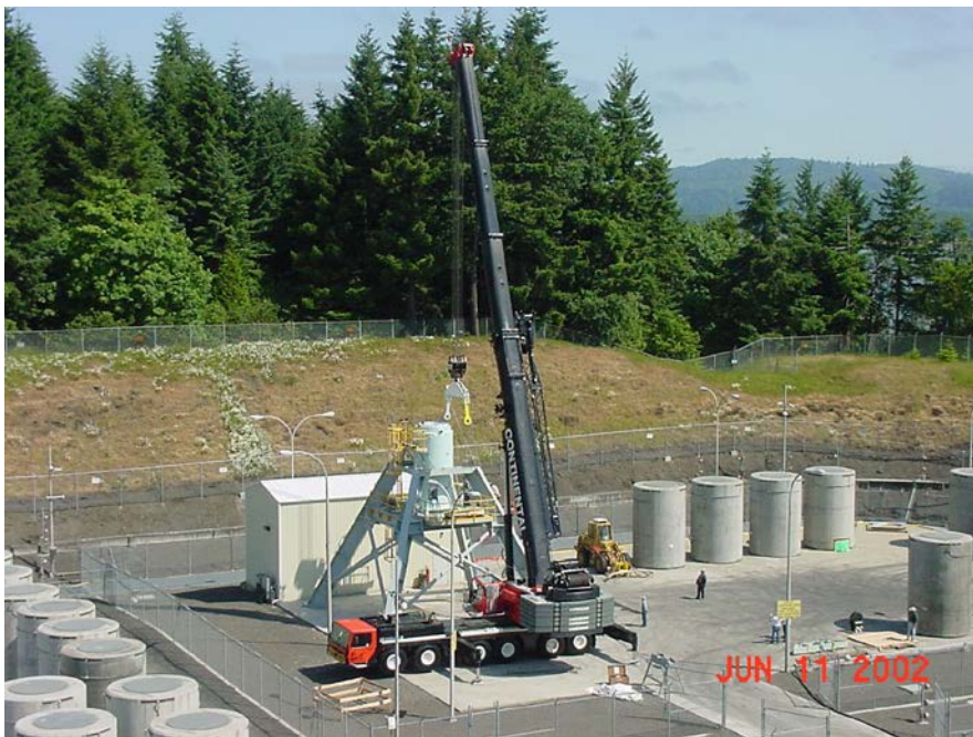
Figure 2-91. Trojan Transfer Station with Transfer Cask and Mobile Crane
