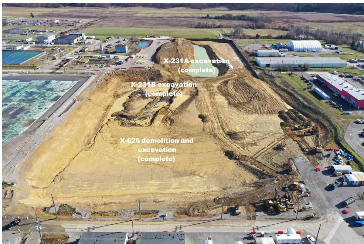
Figure 3.3. Excavation area at the Quadrant I Groundwater Investigative (5-Unit) Area in December 2024 (looking west to east)
