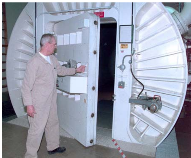
Isolation Door at the Pantex Plant
