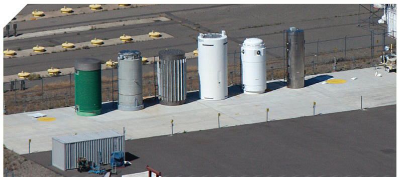
Dry storage casks at the Idaho Nuclear Technology and Engineering Center at Idaho National Laboratory
