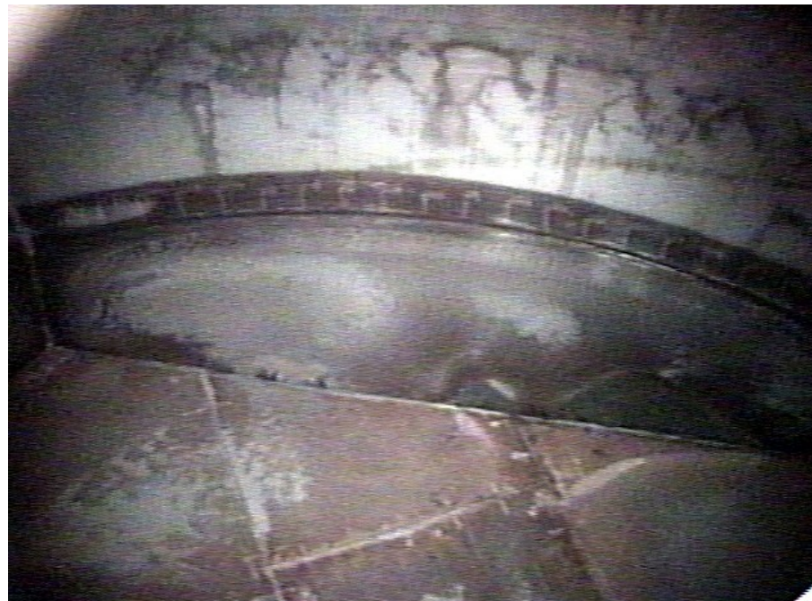
Photo of a previously emptied and cleaned waste tank shows no corrosion issues.
