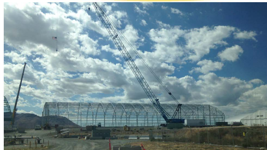
ARP IX retrieval enclosure framing
