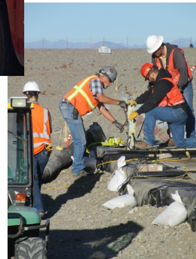
Preparing AMWTP Cargos for Grouting
