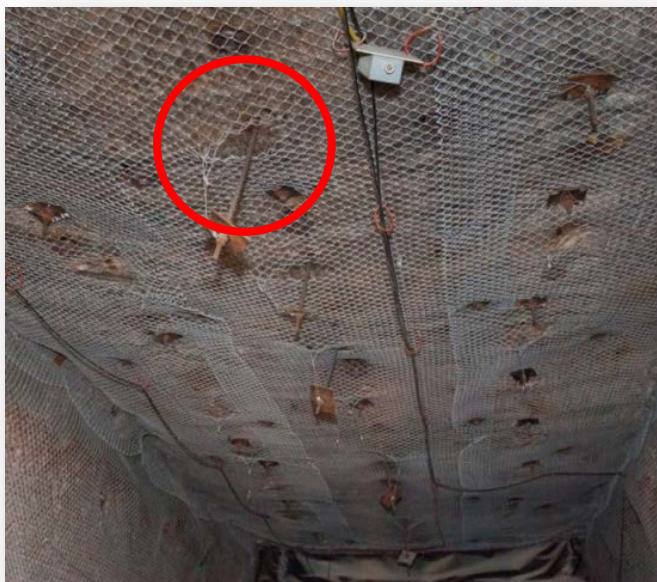
Broken roof bolts
