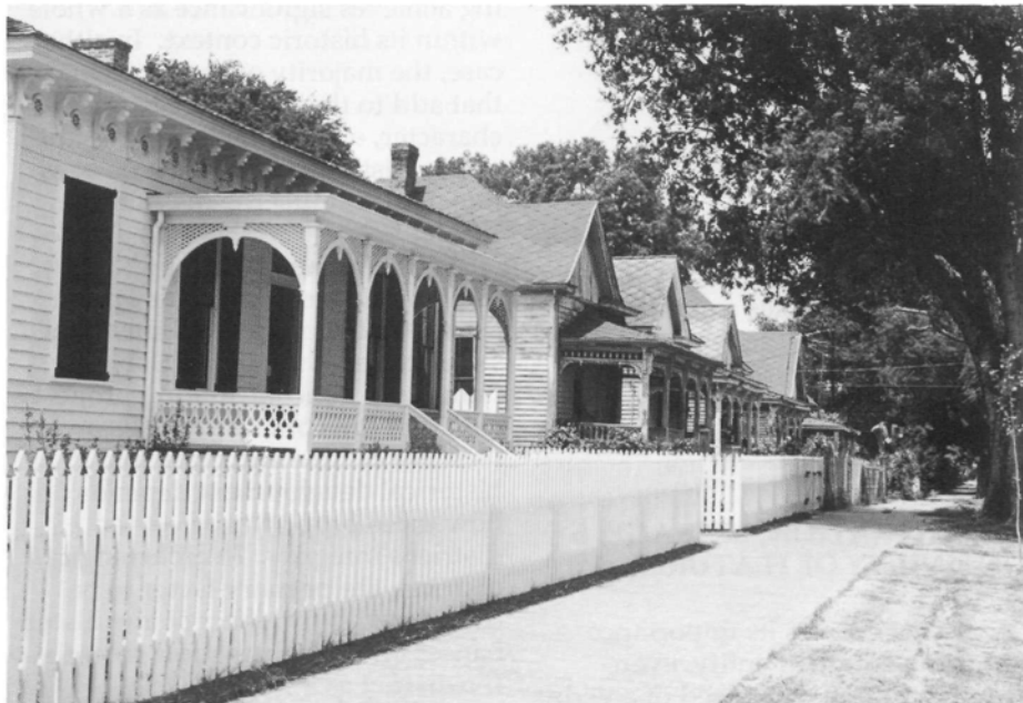
Ordeman-Shaw Historic District, Montgomery, Montgomery County, Alabama. Historic districts derive their identity from the interrelationship of their resources. Part of the defining characteristics of this 19th century residential district in Montgomery, Alabama, is found in the rhythmic pattern of the rows of decorative porches. (Frank L. Thiermonge, III)
