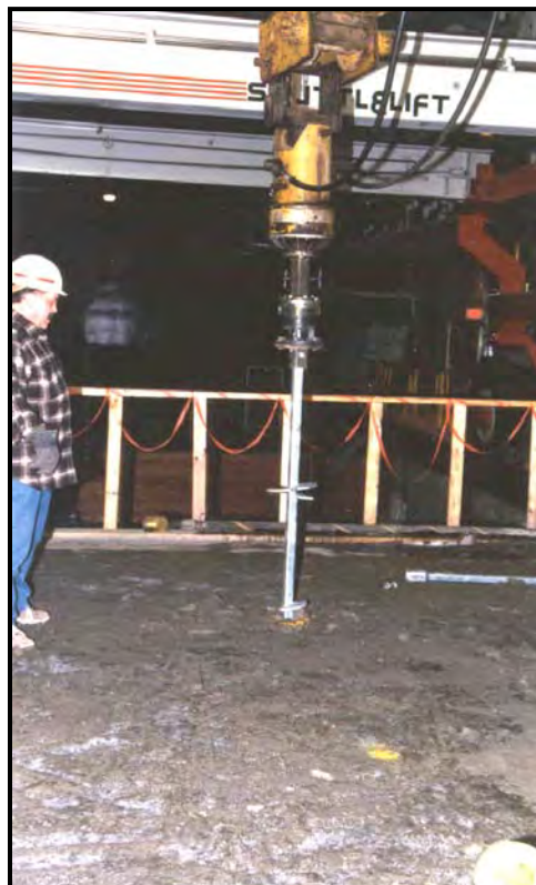
Figure 1.2 Installation of Helical Pier with Excavator and Rotation Head
