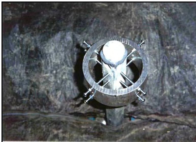
Figure 3.18 Aluminum Collar Bolted to Sides of Pier to Support Arm for Settlement Measurements
