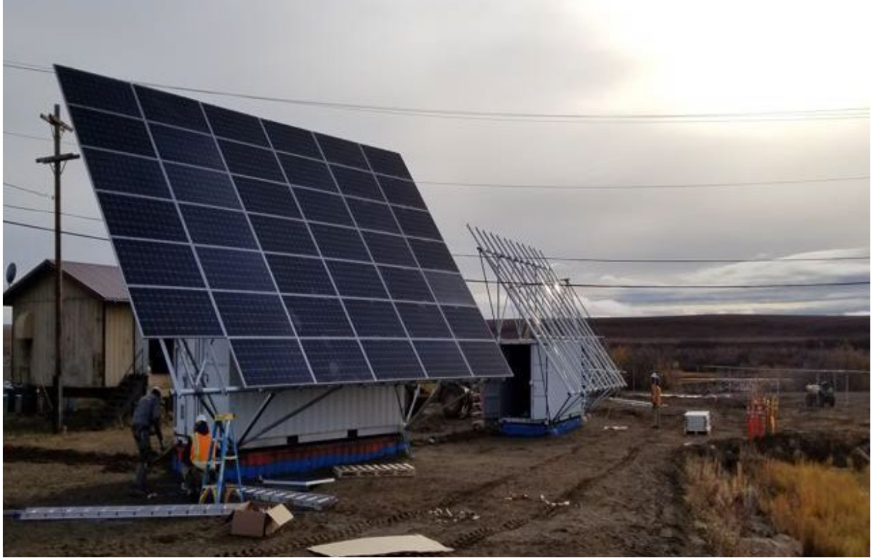
Figure 10 Construction in Progress
