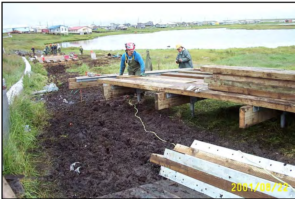
Figure 4.11 Installation of the Boardwalk in Chefnak (VSW)
