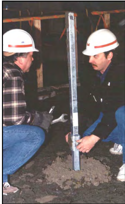
Figure 3.21. Pier Extension is Attached
