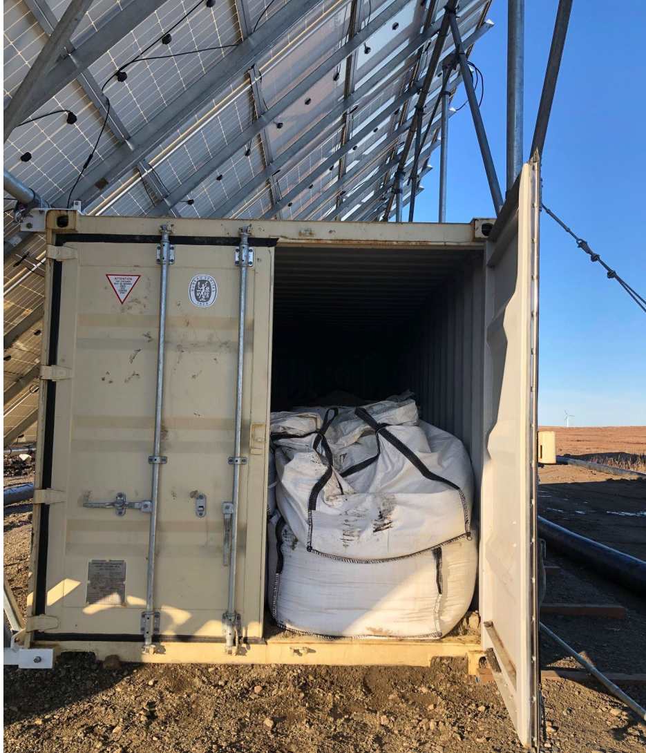
Figure 16 Supersacks filled with gravel to contain ballasting weight inside container
