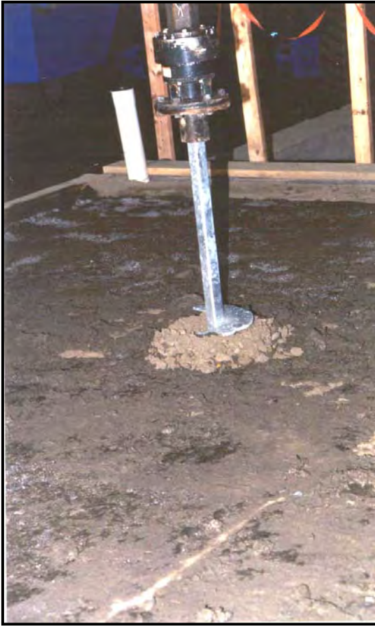
Figure 3.20 Pier Installation
