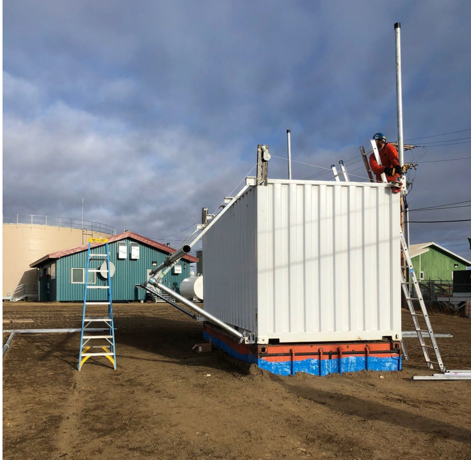
Figure 5 Shipping Container Foundation (Blue Container is Buried)
