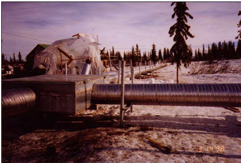
Figure 4.5 Arctic Pipe with Helical Piers as a Foundation in Noorvik, Alaska (ANTHC, DEHE)
