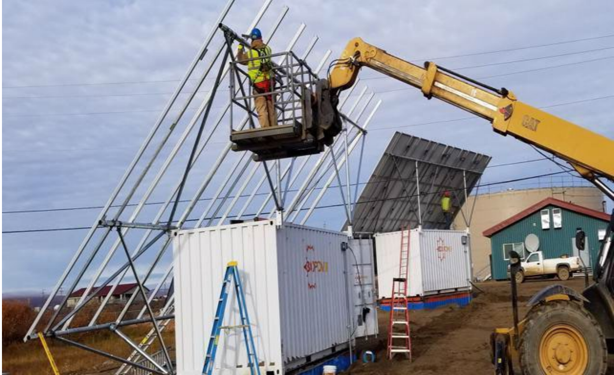
Figure 4 Crew Installing Racking at 45-degree Angle
