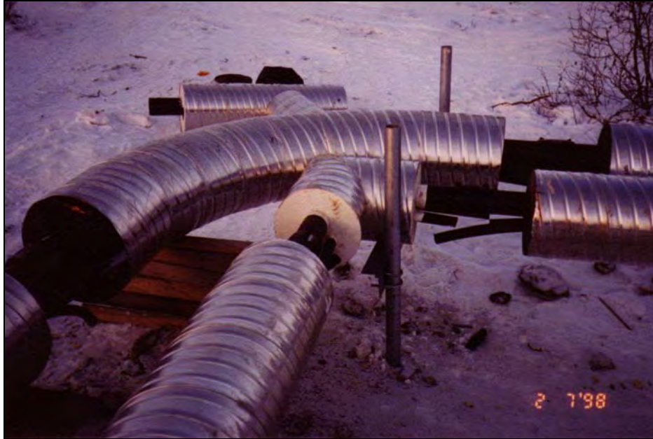
Figure 4.4 Helical Piers in Noorvik, Alaska Installed as Foundations for Arctic Pipe Sewage Installation. The Arctic Pipe Contains a Vacuum Sewage Line. (ANTHC, DEHE)
