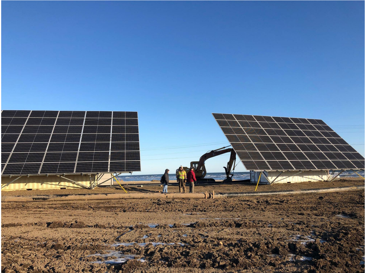
Figure 18 Construction in Progress in Deering
