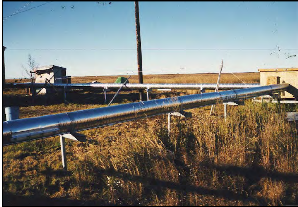
Figure 1.3 Utilidor Supported by Helical Piers in Selawik, Alaska
