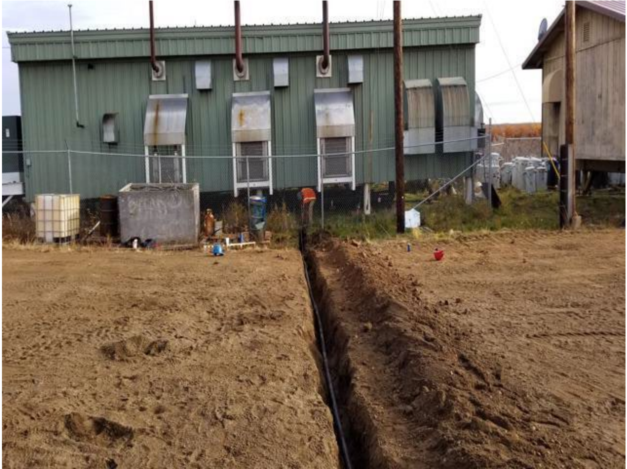
Figure 6 Trenching Conduit and Conductor into Existing Diesel Powerhouse
