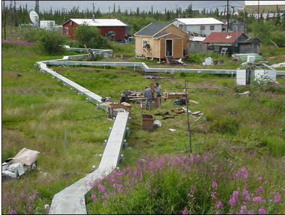
Figure 4.6 Finished Utilidor on Helical Piers in Noorvik, Alaska (ANTHC, DEHE)
