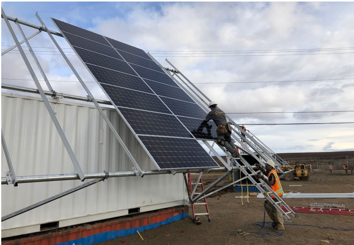
Figure 9 Installing Solar Panels in Buckland
