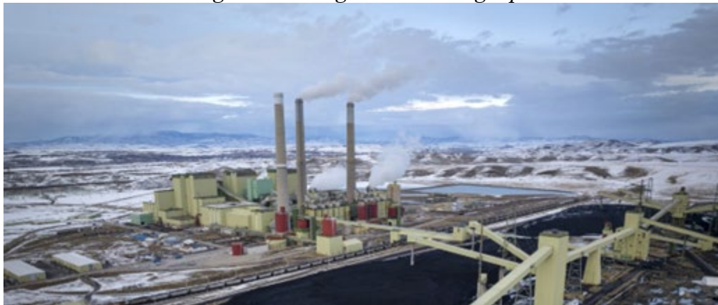
Figure 8: Craig Plant Photograph
