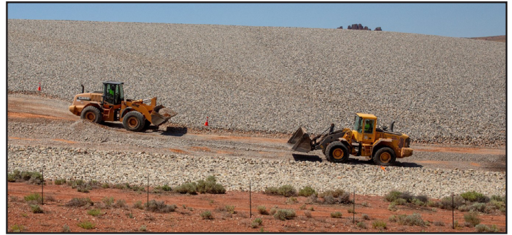
Mexican Hat disposal cell during the interim cover protection project.
