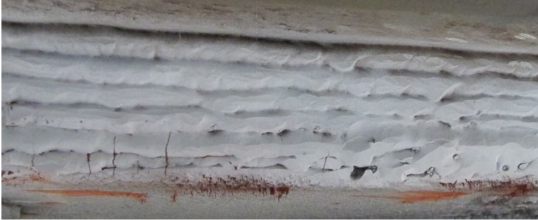
Figure 11. Cracks in B-end tri-span bolster, C-truck centerplate
