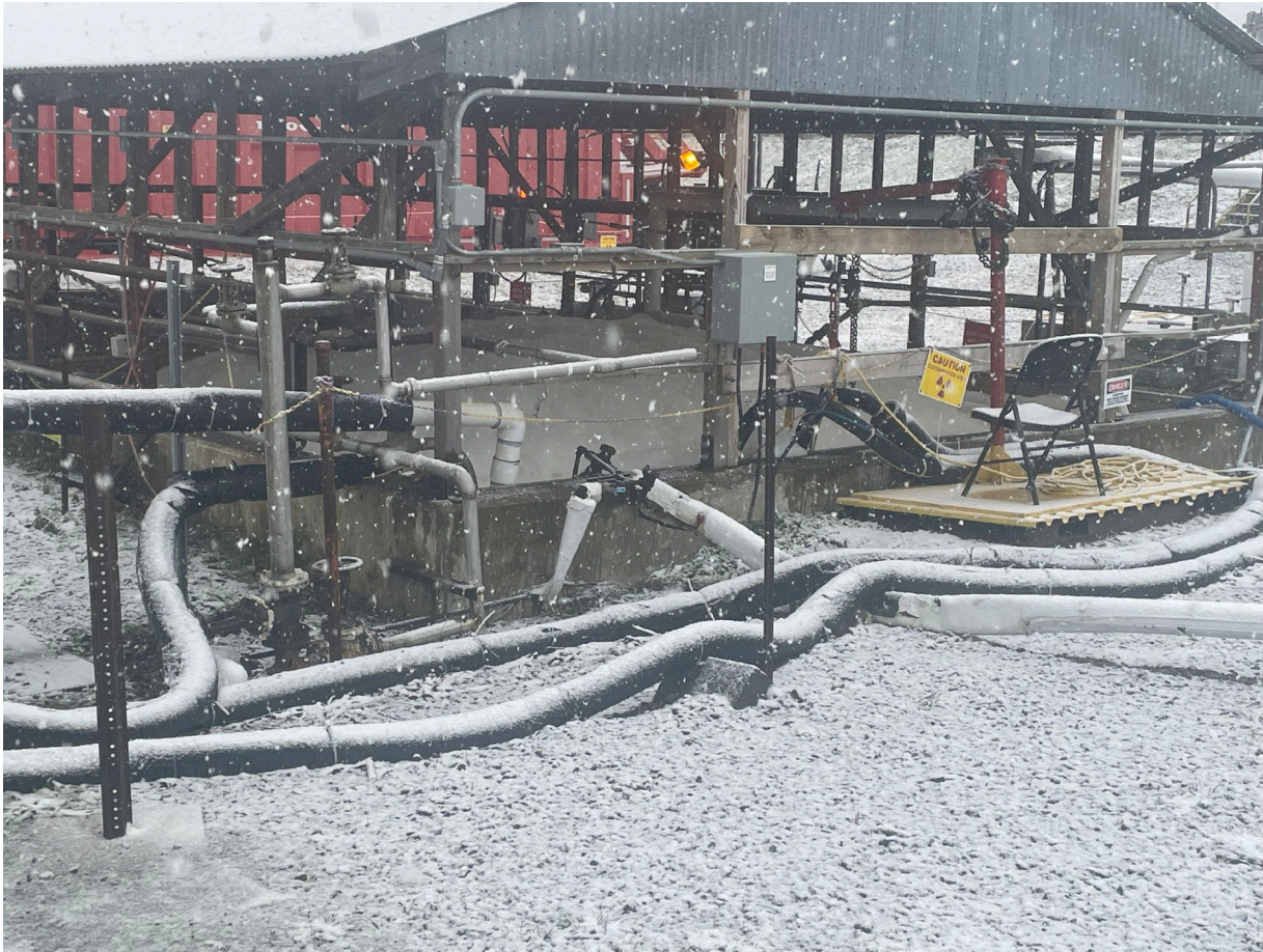
Stormwater Interceptor System Designed to Handle Precipitation and Dust-Suppression Flows During All Weather Conditions
