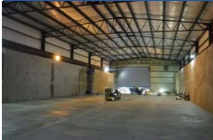
New concrete floor inside Drum Cell
