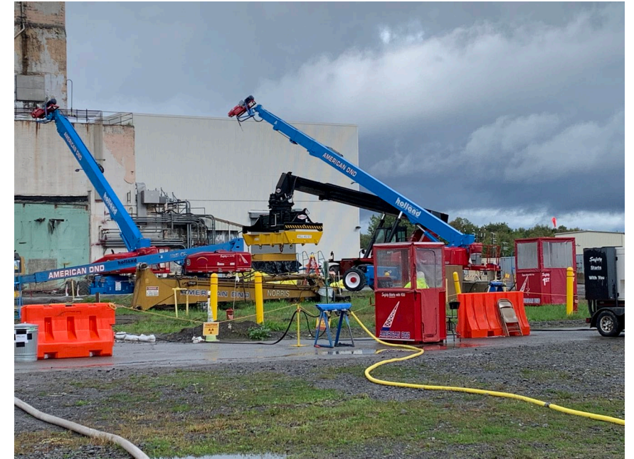
Remotely Operated Turbine High Lift Sprayers
