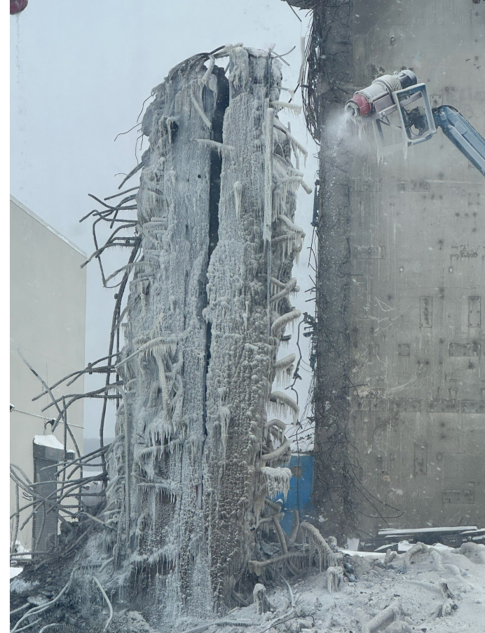
Application of Fixative (Gorilla Shot) Lock Down of Soils and Debris at Shift End
