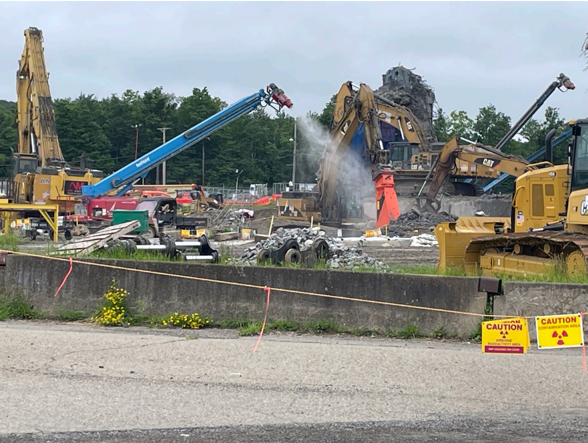
Dust Suppression During Equipment Moves and End Effector Changes Minimized Ancillary Dust
