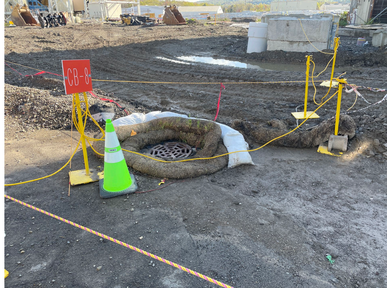
Catch Basins Outfitted with Sediment Controls and Internal Filter Socks Routinely Inspected, Surveyed, and Cleaned
