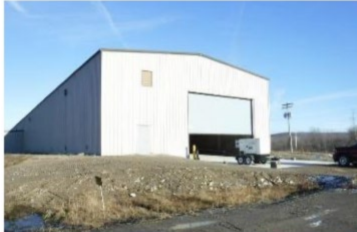
Drum Cell – New rollup door and driveway
