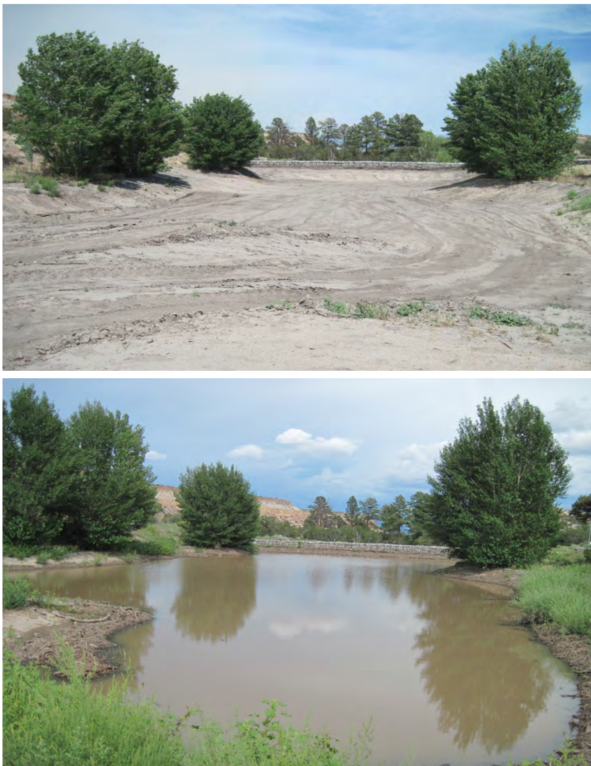
Figure 7-15 Los Alamos Canyon weir before (top photo) and after (bottom photo) storm-water flows
