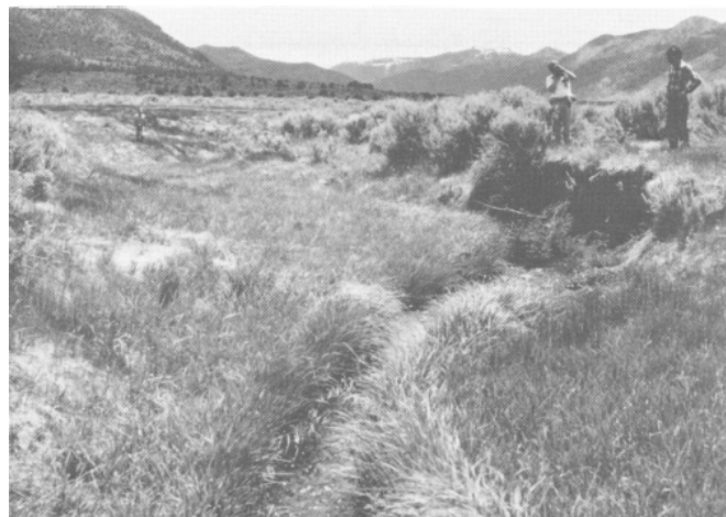
Figure 5 – Gullies that are old, wide, and well managed become valued again for riparian vegetation, fish, and wildlife habitat, water and sediment storage, and aesthetics.
