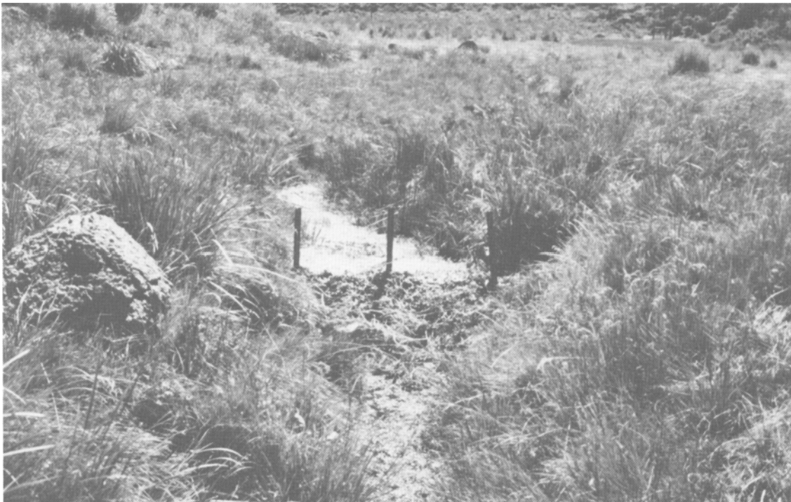
Figure 6 — Single fence rock-check dam, Clark Canyon, California, August 4, 1987.
