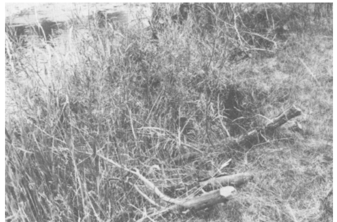
Figure 3 — Juniper revetment 8 years after placement. Trees were sodded in and barely visible.
