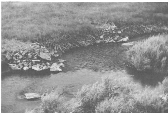
Figure 4 - Juniper revetment used in combination with rock deflectors.
