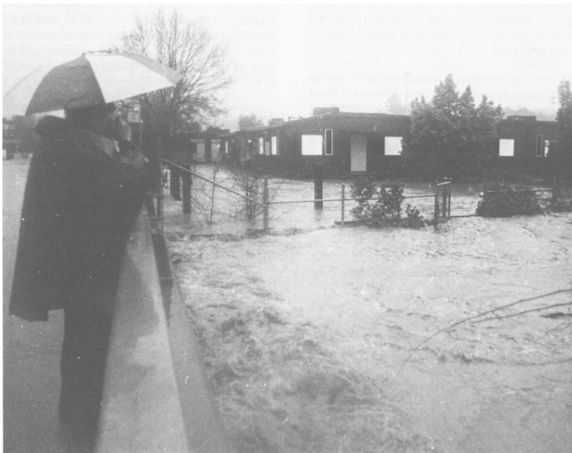
Figure 1 — Corte Madera Creek during the January 4, 1982 flood overtopping its banks just upstream of a bridge near the College of Marin. Turbulence in foreground is water hitting the bridge face. The rectangular concrete channel is about 2 feet below water surface during a 15-year recurrence flood of 4,500 cfs. The channel was designed to contain a 200-year flood of 7,800 cfs with 2 feet of freeboard. Similar flooding occurred in February of 1986. (Photo: Philip Williams)
