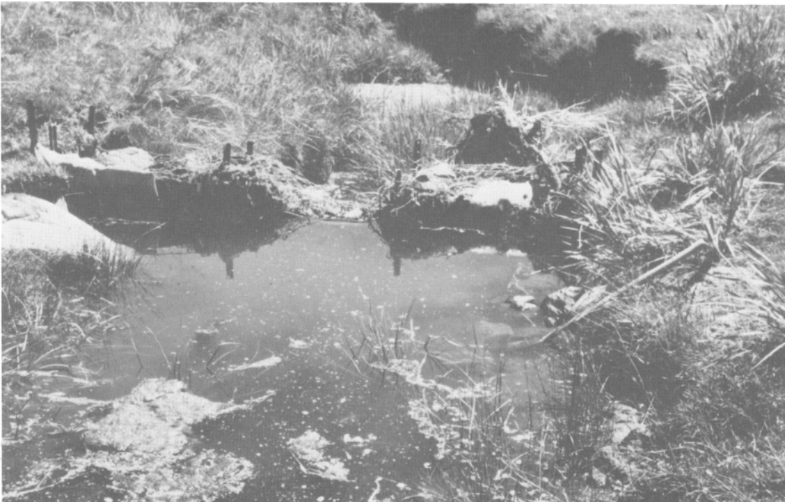
Figure 4 - Same gabion basket structure as in Figure 3 after modification and lining, Clark Canyon, California, July 17, 1986.
