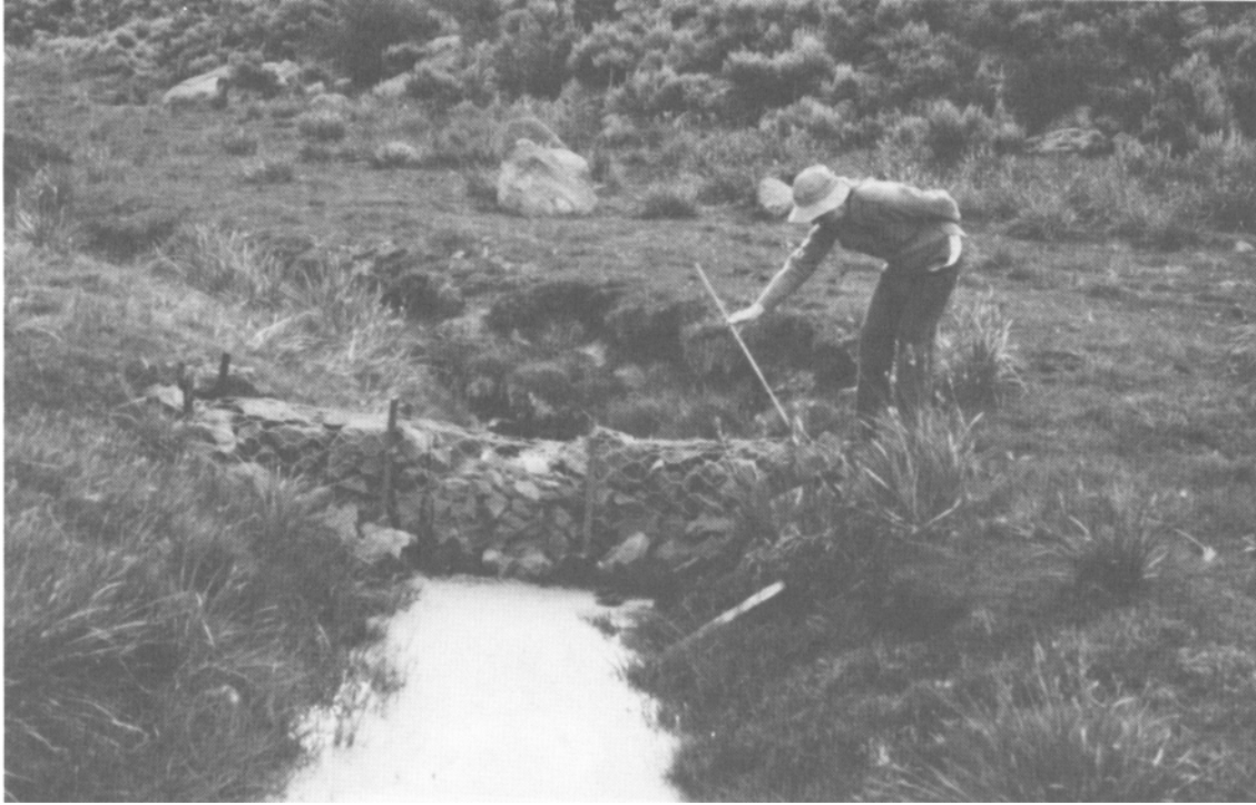
Figure 3 - Unlined gabion basket structure, Clark Canyon, California, July 28, 1984.
