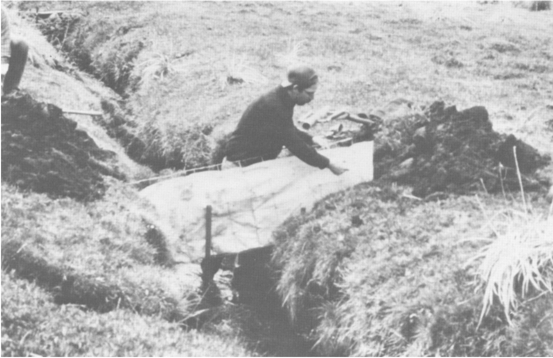
Figure 5 — Installation of single fence rock-check dam, Clark Canyon, California, October 10, 1985.
