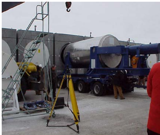
Loading a DSC into a Horizontal Storage Module at the TMI-2 ISFSI
