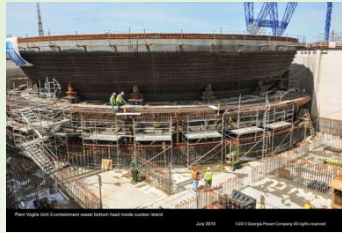
Vogtle Unit 3 CVBH in place and cooling tower under construction (Courtesy of Southern Company)
