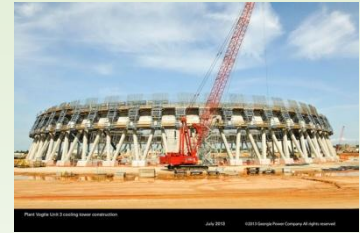
Vogtle Unit 3 CVBH in place and cooling tower under construction (Courtesy of Southern Company)
