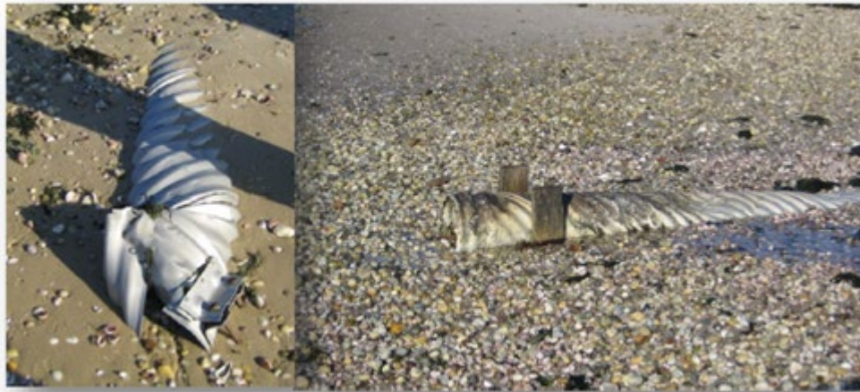
Figure C.2.10 - Culverts, pipes adjacent to Shinnecock Indian Cemetery. Pipes are clogged, and in need of repair.
