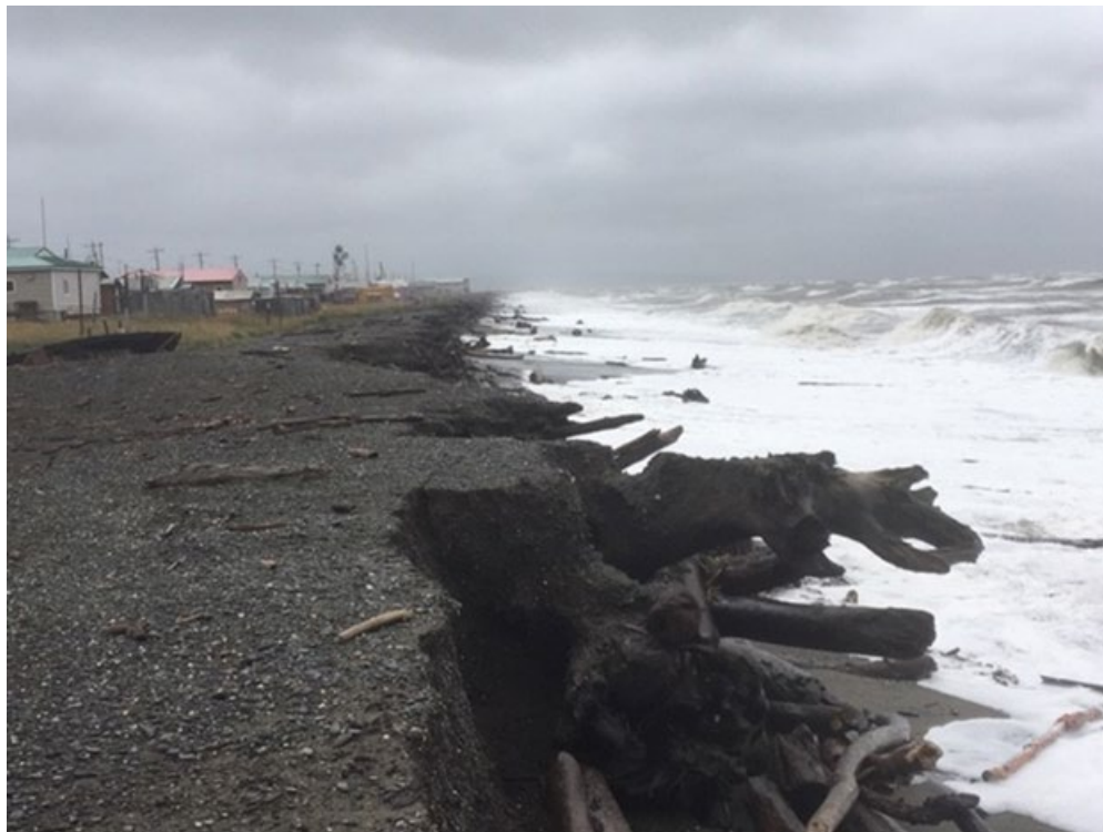
Figure 5. On August 2, 2019, an unusual summer storm washed 350,000 cubic feet of Shaktolik's storm surge berm into the Bering Sea, leaving all of the community's infrastructure highly vulnerable to fall storms (shown above). Shaktolik must apply to a myriad grant programs across many different state and federal agencies to secure funding to respond to their threat. Credit: Sophia Katchatag, Native Village of Shaktolik.
