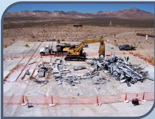
Demolition of the movable shed and nuclear furnace piping at NTS Test Cell C Facility.
