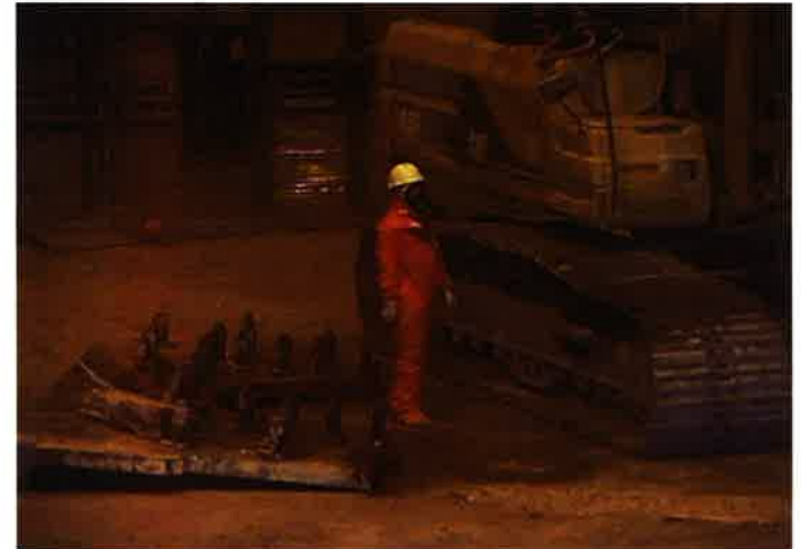
Lower thermal shield plate removal from the MTR reactor vessel
