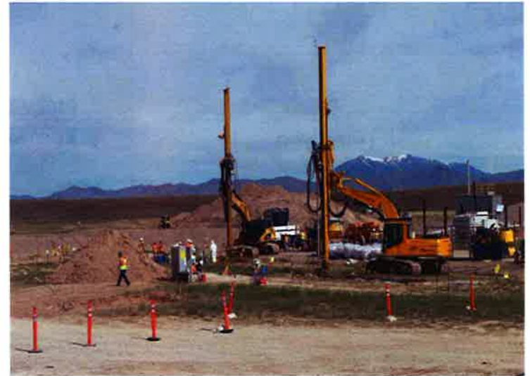
In-situ grouting rigs
