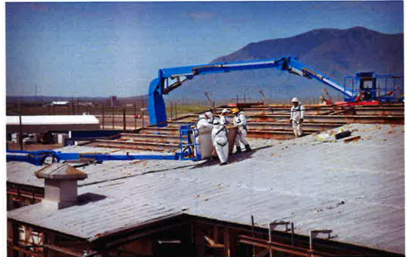
CPP- 601 transite removal and steel-structure demolition
