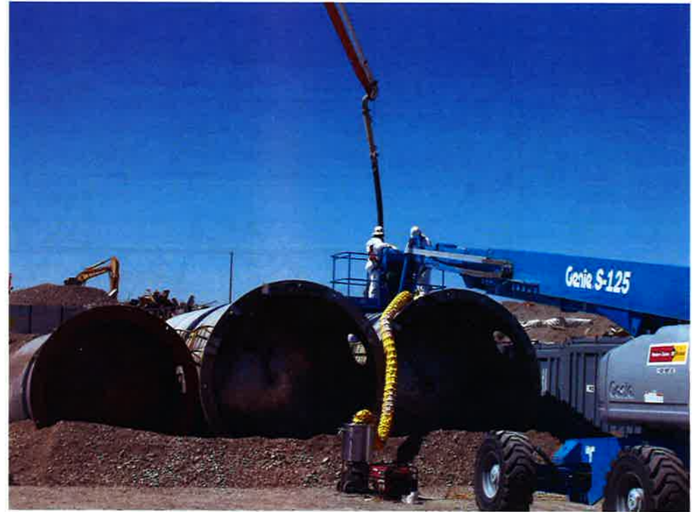
Grouting Tank Farm CPP-694 tanks
