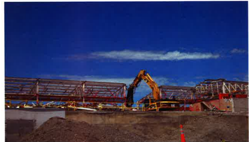
CPP- 601 transite removal and steel-structure demolition
