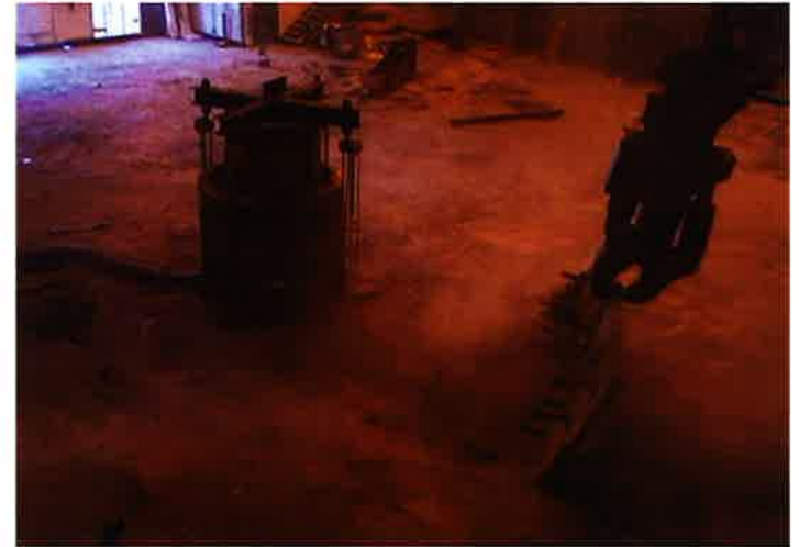
Lower thermal shield plate removal from the MTR reactor vessel
