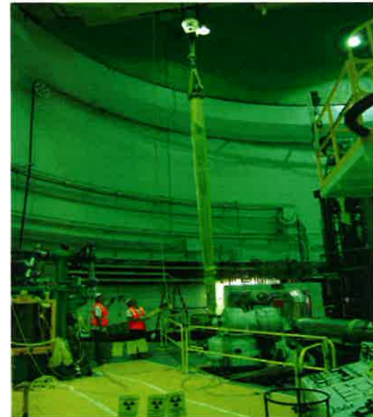
MFC-767 Reactor vessel nozzle removal: Camera inspections
