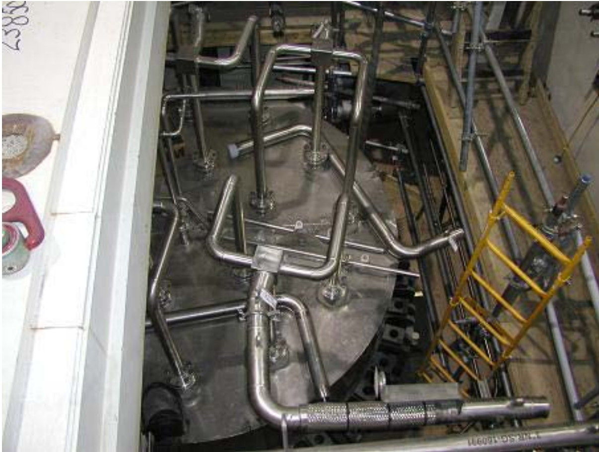
Top of Process Gas Filter in 4-Pack Cell
