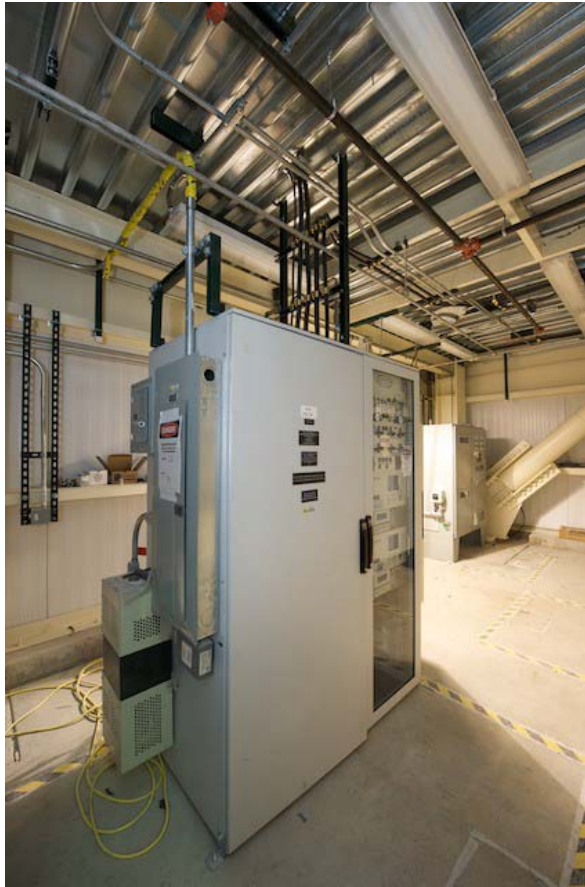
Off-Gas System Continuous Emissions Monitor Panel
