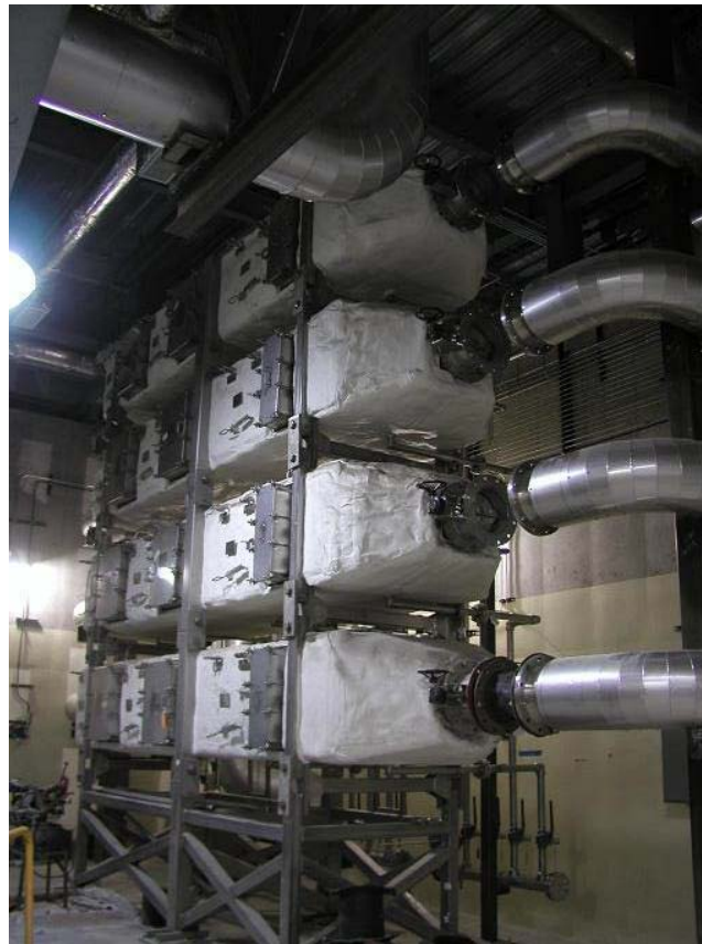
Off-Gas System HEPA Filter Bank
