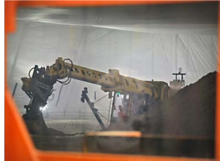
Exhumation and sorting of waste from Pit 9 (ARP-V)
