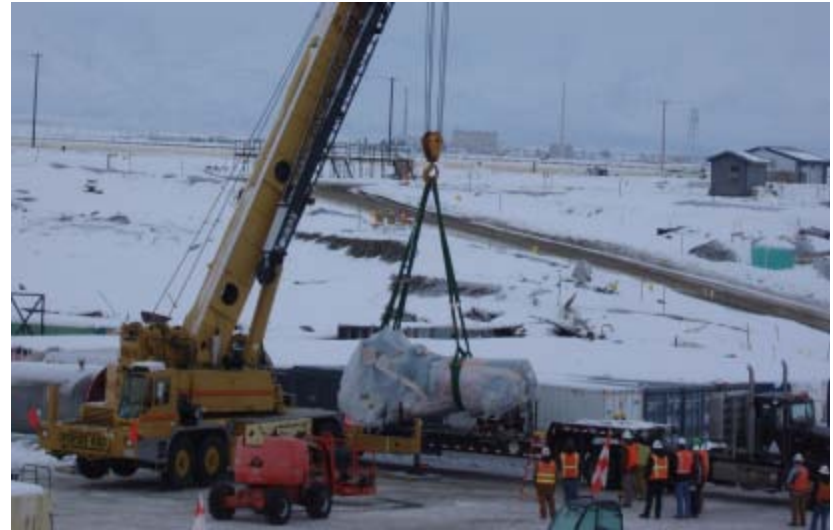
MTR Reactor vessel transportation to ICDF
