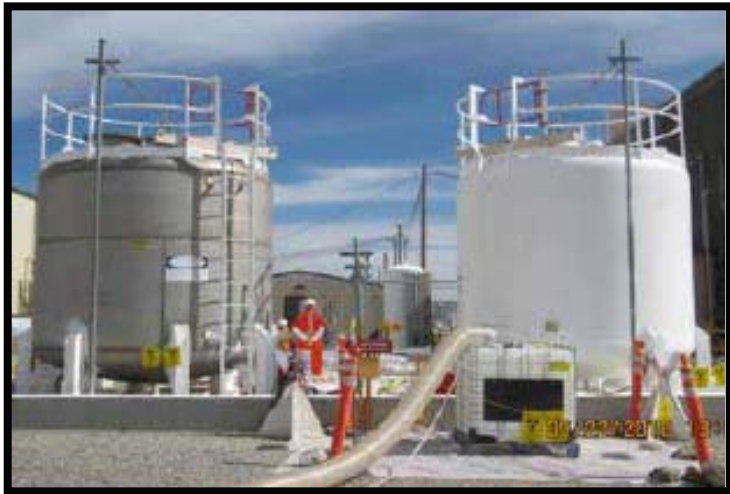
Contents of Alcohol tanks removed (MFC-793A)
