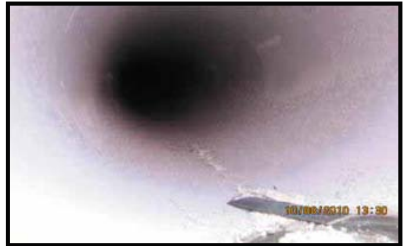
Passivated sodium inside the secondary sodium yard piping
