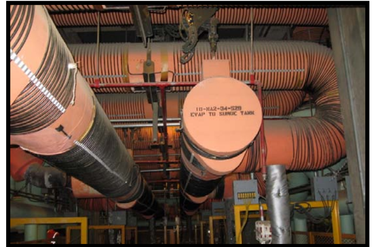
Asbestos covered piping in MFC -766 before removal
