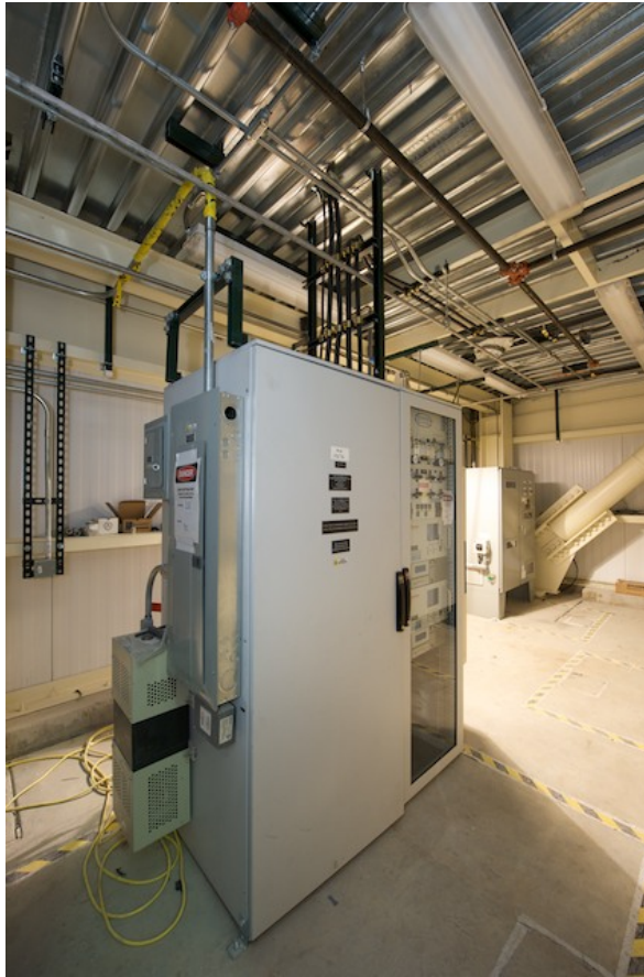
Off-Gas System Continuous Emissions Monitor Panel
