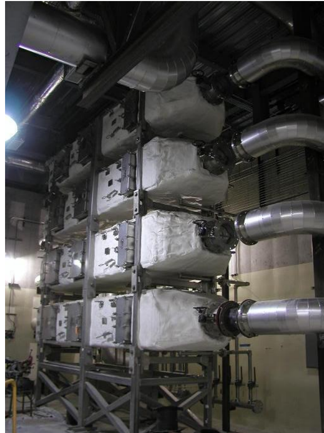
Off-Gas System HEPA Filter Bank
