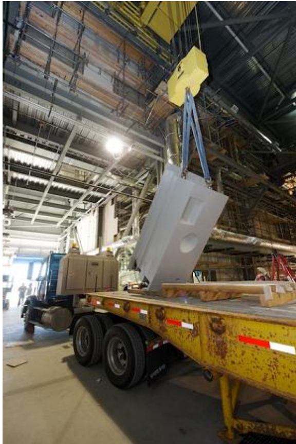
Unloading of Process Cell Shield Door
