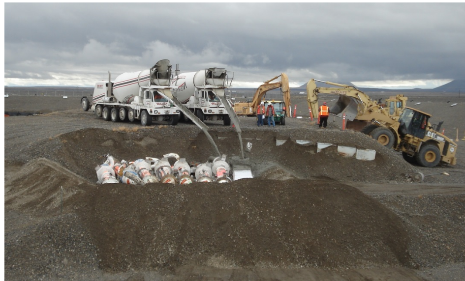
Flood grouting of MFC heat exchangers November, 2015
