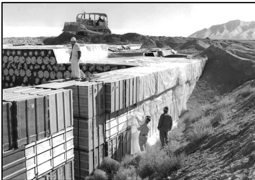
TRU waste was piled on plywood and covered with dirt (left), or stored in a non-compliant air support building (below)
