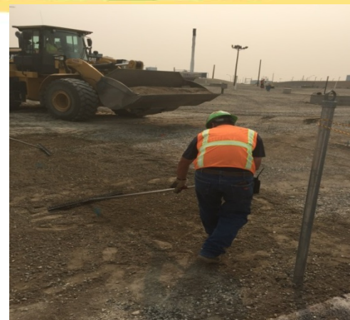
Placing crushed base material on north end of Tank Farm in preparation for asphalt
