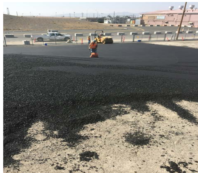
Placing asphalt on berm, south west side of Tank Farm
