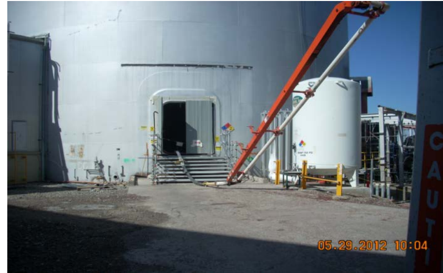
Grouting primary tank annulus
