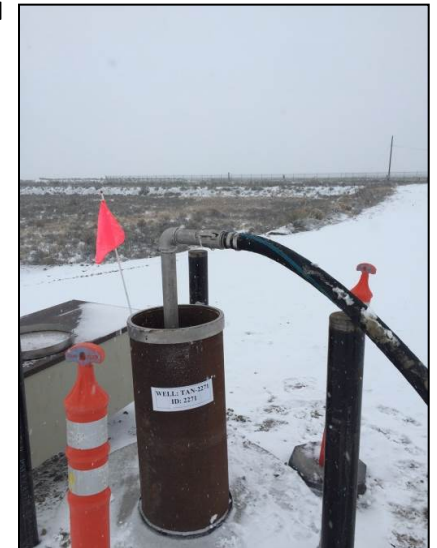
ISB Treatment Injection into TAN-2271
